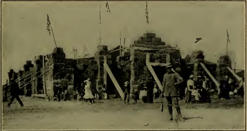
FIG. 68. Temporary county fair building constructed of baled alfalfa hay. In a pioneer section.
