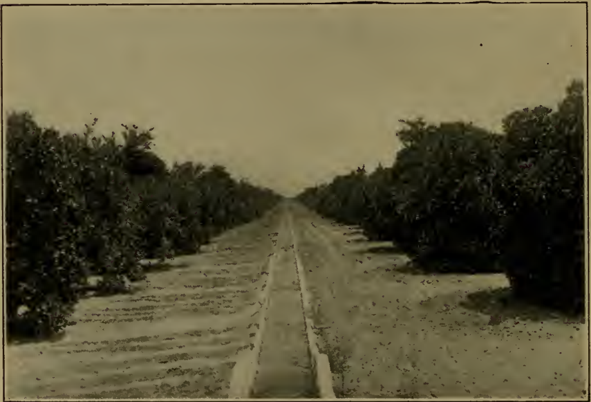
FIG. 34. A permanent ditch in an orange grove (Redlands).
