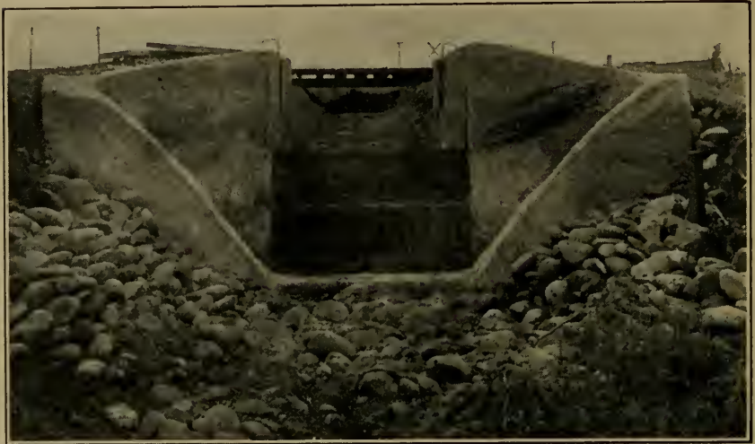
FIG. 135. Concrete drop in ditch.
