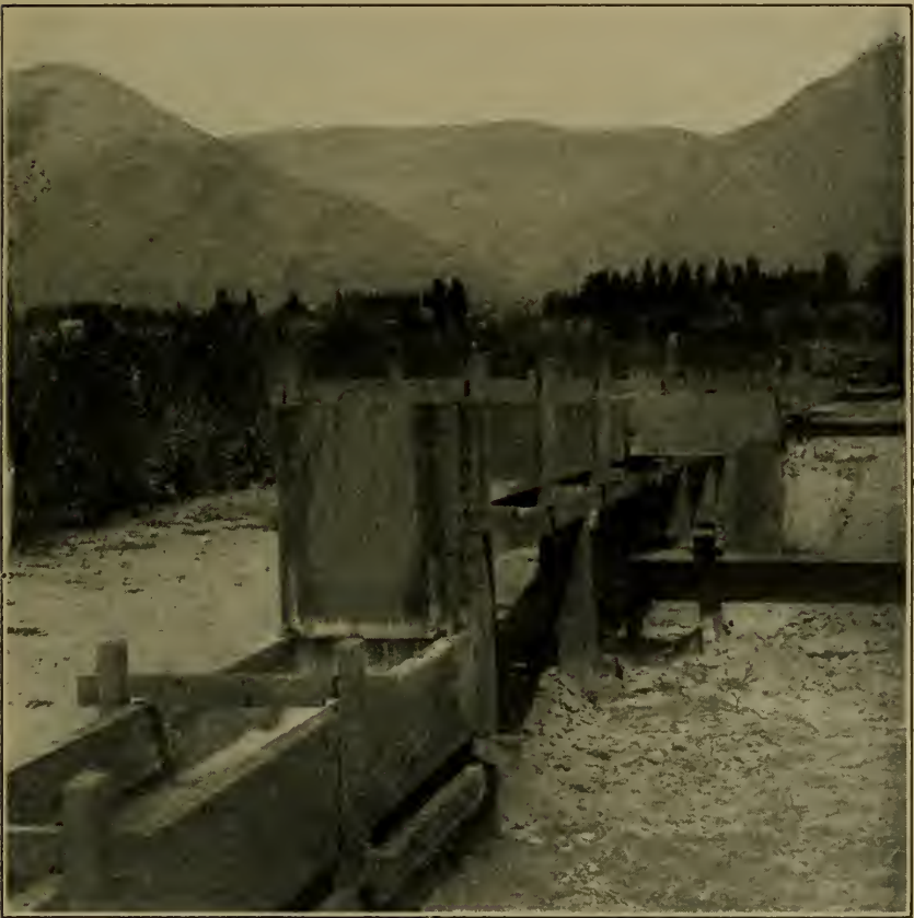
FIG. 136. Drop in flume.
