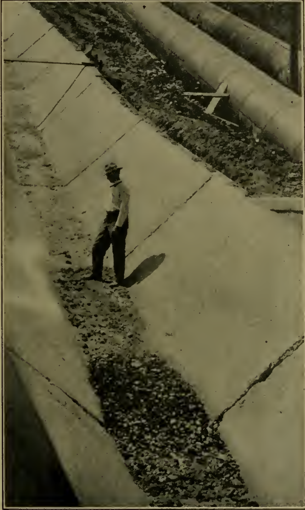
FIG. 109. Lateral lined with concrete.
