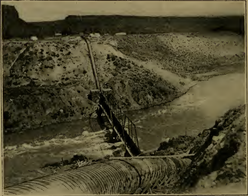
FIG. 91. Canal crossing river in an inverted syphon.
