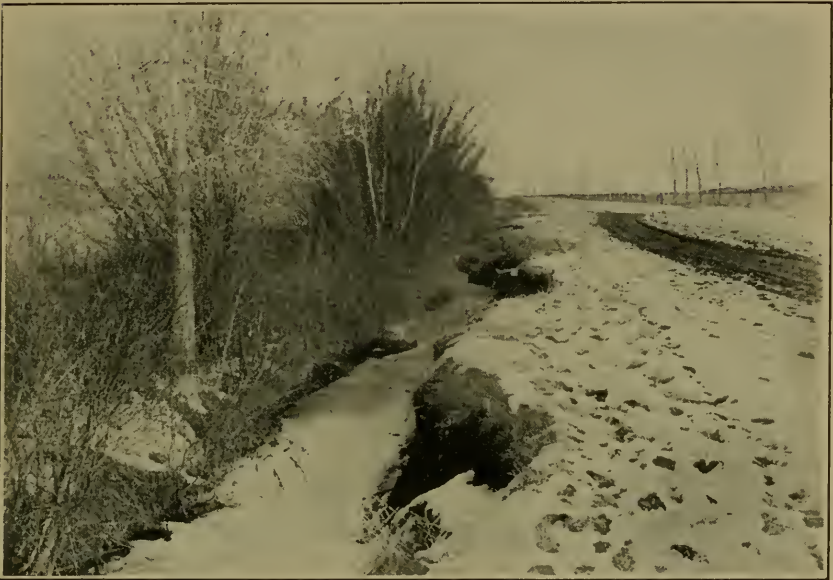
FIG. 18. Badly corroded ditch due to excessive fall. On a larger scale this is the action of swift rivers.
