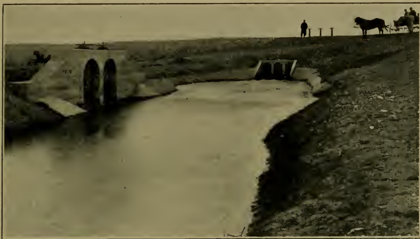
FIG. 93. Lateral outtake from large canal.
