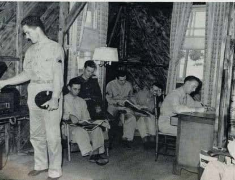
Signal Company day room.
