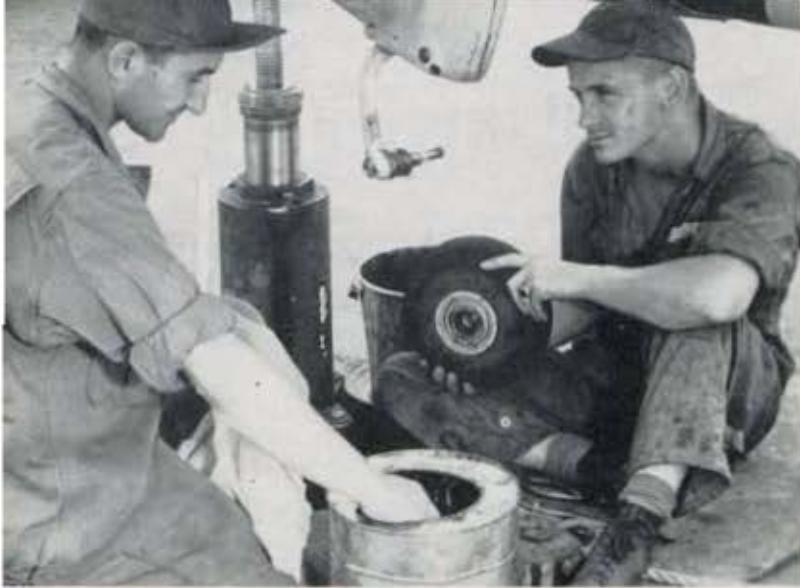
Re-packing a tail wheel.
