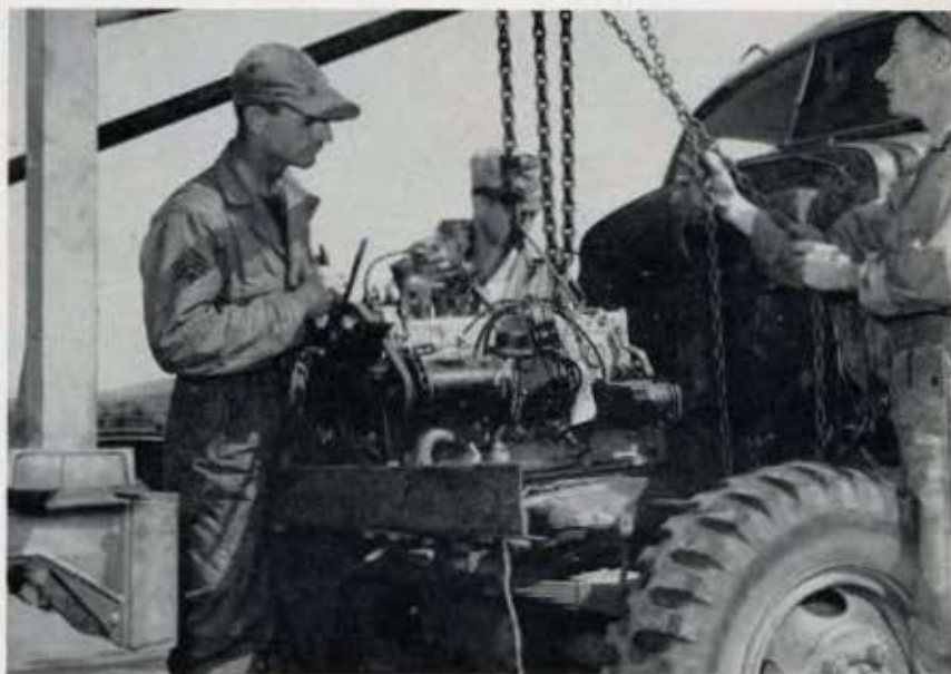
Pulling out a truck motor.
