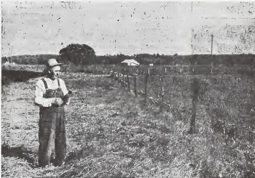
NOT FIGURED IN THE LOSS —Harold Mooney, Sr., is shown repairing his fences following the September 13 flood. Such repairs must be made immediately to keep livestock in lots and pastures. Mooney, who has led the steering committee in the move to get the watershed on Middle Creek, estimates it will cost him between $1,000 and $1,200 in materials and labor to fix the fences washed out by the flood. He was born and reared on this Middle Creek valley farm and reports the water was five inches higher than in any previous flood he can recall—in slightly over fifty years. Such fence damage is not estimated in the loss of crops, roads and other property hit by the flood. (Soil Conservation Service Photo)
