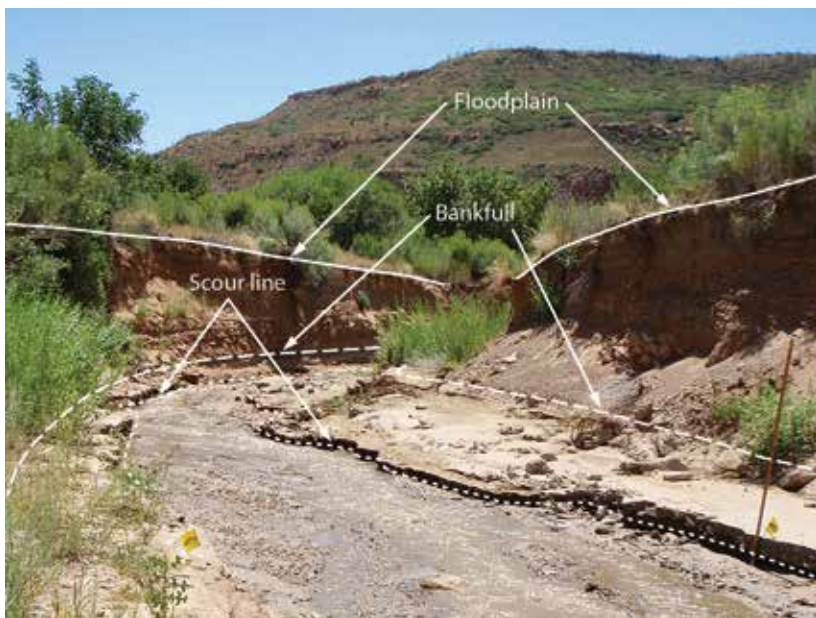
Figure D6. Location of bankfull, floodplain, and scour line heights. Bankfull and floodplain heights differ when no flat depositional feature exists at bankfull height.
