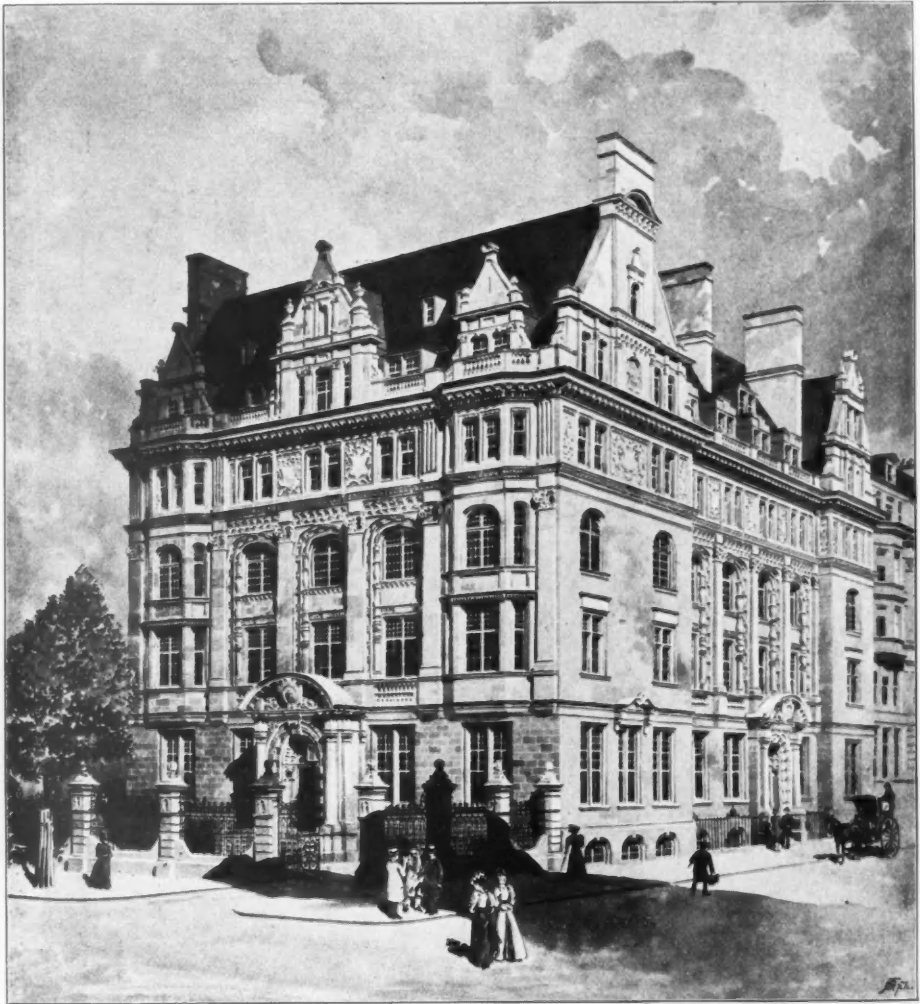
Hamilton House, Victoria Embankment, for the Employers' Liability Corporation, Ltd., WILLIAM EMERSON, P.R.I.B.A., Architect.
