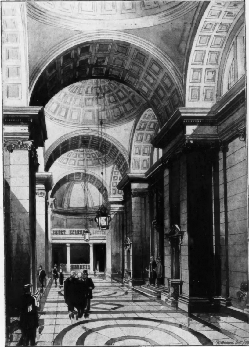
1728. New States Hall, Guernsey, Interior of Salle d'attente , EDWARD W. MOUNTFORD, F.R.I.B.A., Architect (For Perspective View and Plan, see Vol. 15, pp. 60, 61.)
