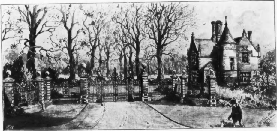
Lodge and Entrance Gates, Childwick Bury, St. Albans, ROBERT W. EDIS, F.S.A., Architect.
