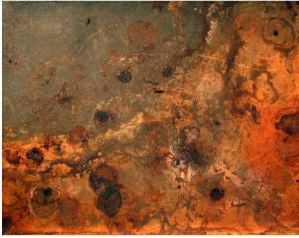
• Figure 1381 Rust Texture
