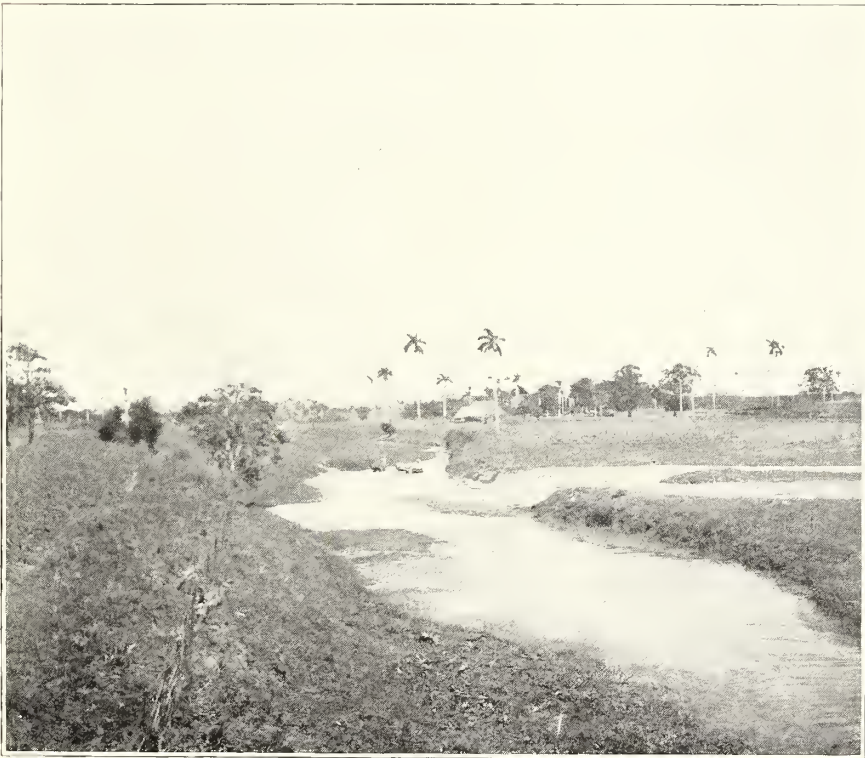
RIO DEL PINAR, LOOKING UPSTREAM FROM BRIDGE.
