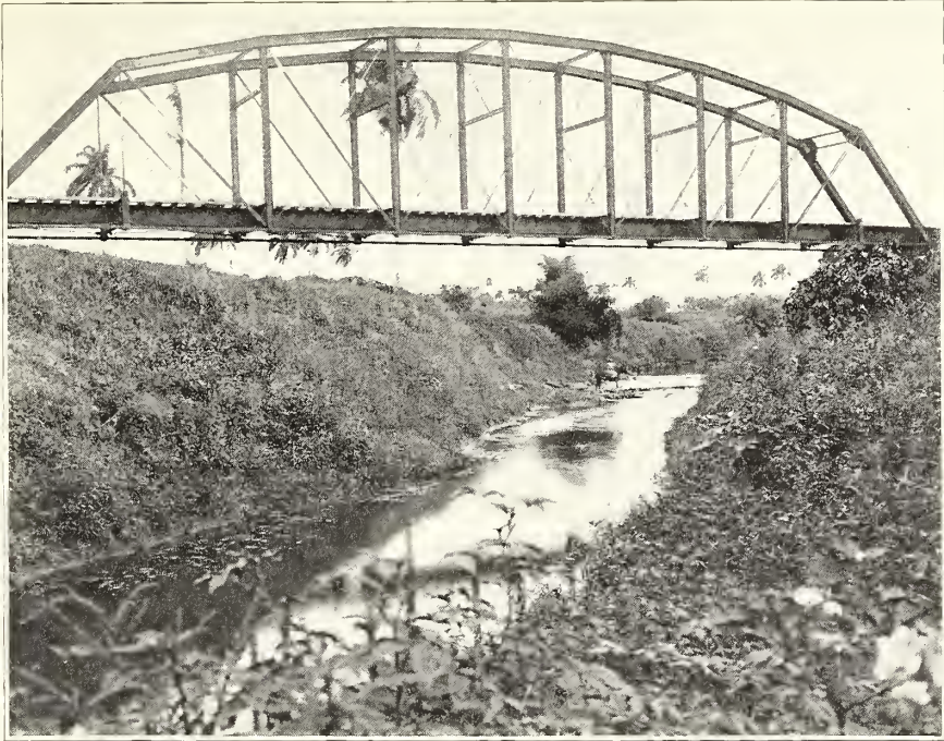
RIO SAN DIEGO AT PASO REAL, LOOKING UPSTREAM FROM BELOW WESTERN RAILROAD BRIDGE.
