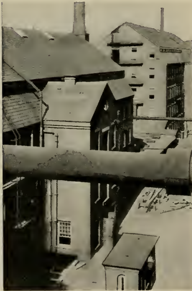
OLD MILLS AND SPRINKLER FEEDERS
