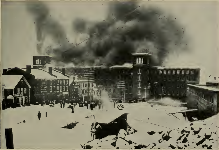
VIEW OF COCHECO MILL, SHOWING FIRE IN PROGRESS
