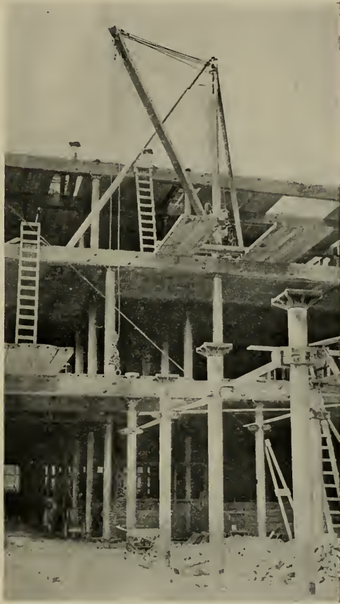
PLANK AND TIMBER IN CONSTRUCTION SHOWING CAST-IRON COLUMNS AND PINTLES
