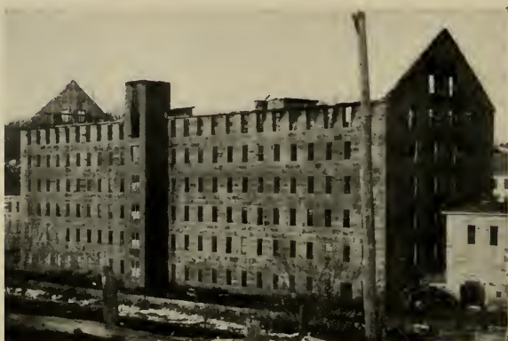
OLD STEEP ROOF BURNED OFF
