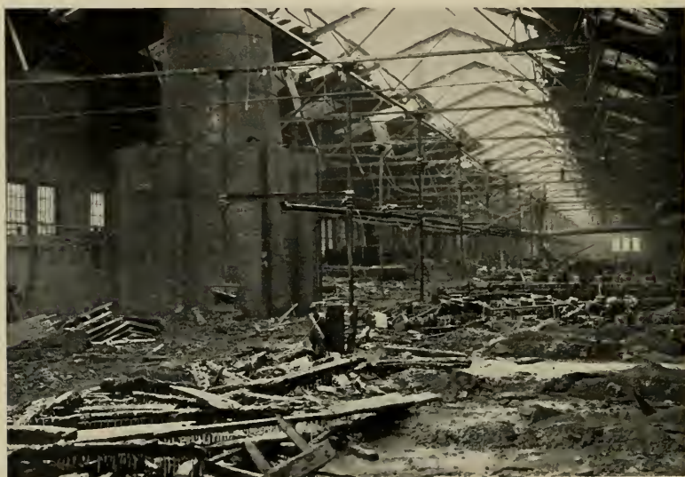
FIRE IN UNSPRINKLED FOUNDRY ROOF, EXTINGUISHED BY HOSE STREAMS GOULD COUPLER CO.
