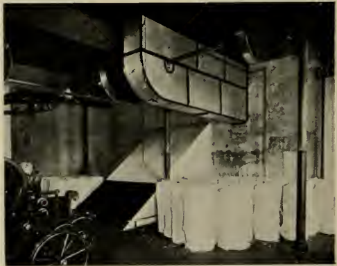
SLOPING CEMENT ENCLOSURE AT FLOOR. METAL BOXING AT CEILING
