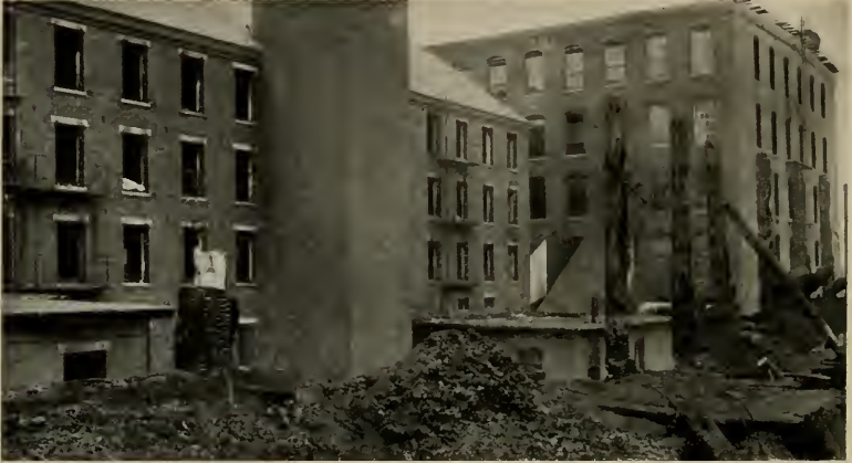
EXTERIOR OF PICKER HOUSE AT LEFT, SHOWING BURNED OUT WINDOWS, AND MILL AT RIGHT WITH BURNED CORNICE AND END WINDOWS ALSO BURNED OUT
