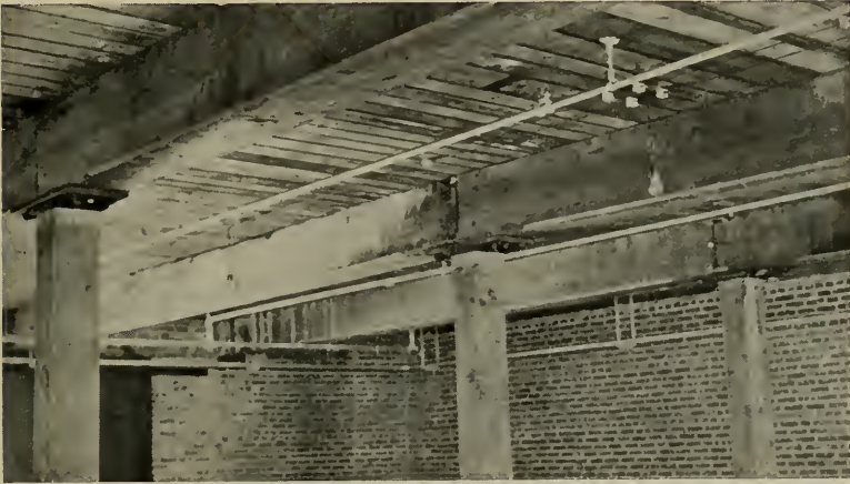
PLANK AND TIMBER CONSTRUCTION
