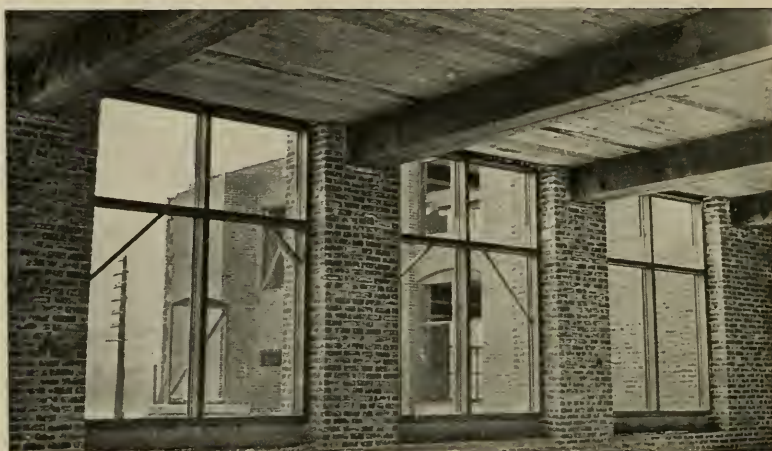
PLANK AND TIMBERS WITH DOUBLE BEAMS
