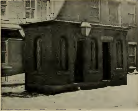
EXTERIOR OF VALVE HOUSE
