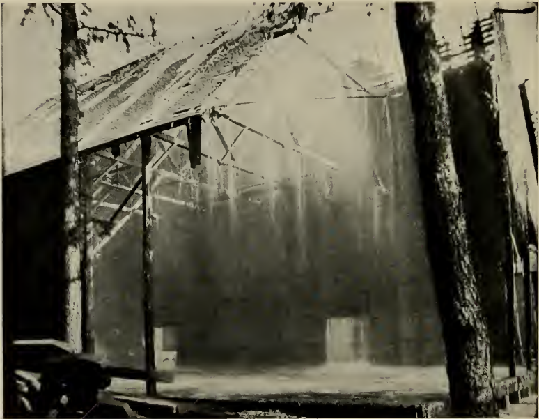
NASHUA STOREHOUSE, SHOWING THE DELUGING DISCHARGE FROM SEVENTY-FIVE OPEN SPRINKLERS
