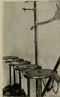
INTERIOR OF VALVE HOUSE
