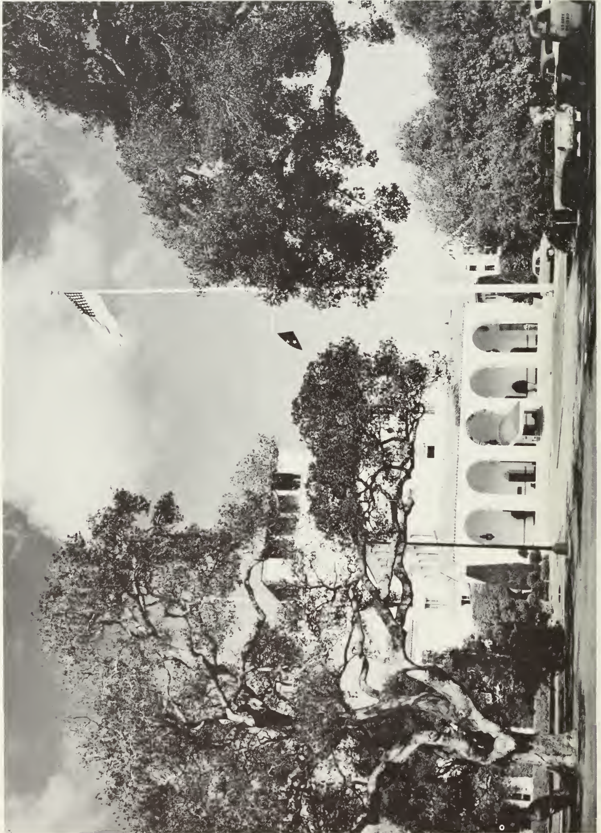
Herrmann Hall, the Administration Building. This building contains the offices of the Superintendent, the Academic Dean, and the Administrative Command. The wings, extending toward the west, contain the General Line and Naval Science School, and the Bachelor Officers' Quarters.
