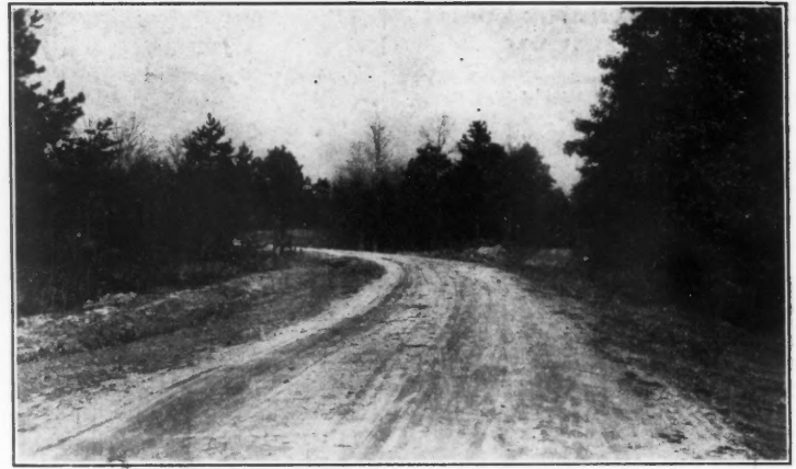
Where traffic does not warrant the heavy expense of a concrete or asphaltic road, the community is served by hard-surface and sand-clay roads, which are frequently scraped, rolled, and resurfaced by the state maintenance corps.
