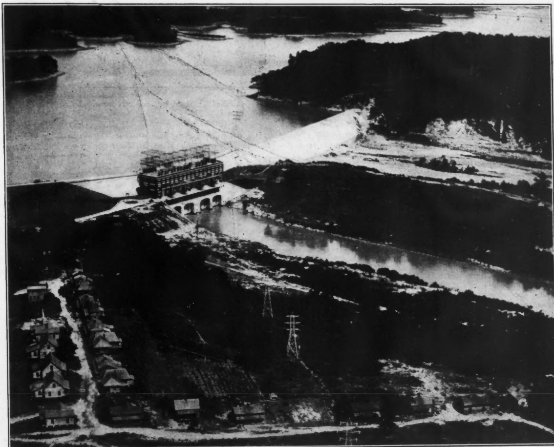
Development of the state's great latent water powers has been an important factor in the growth of the textile industry in recent years. Above is one of the newest hydro-electric plants of the Southern Power Company on the Catawba River. This installation can generate 80,000 horse-power.
