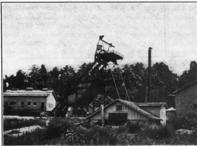
GENERAL VIEW OF HEADFRAME AND SURFACE PLANT, FRENCH CREEK MINE
