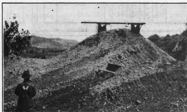
Fig. 47—Returning empty scraper. Note method of hanging sheave blocks from scaffolding that has been built on the edge of embankment.
