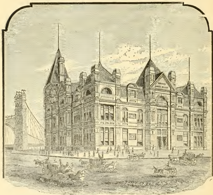
THE UNION DEPOT. (IN PROCESS OF ERECTION.)
