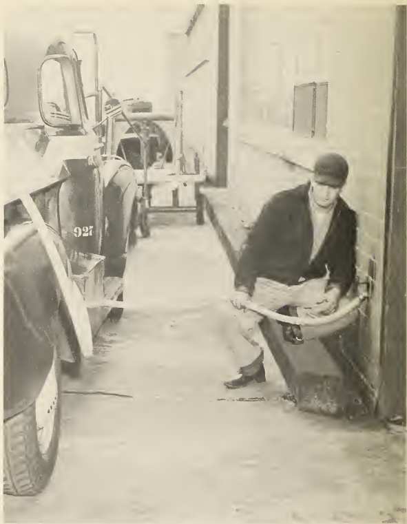
Filling water truck. (Note downward-directed hydrant outlet.)
