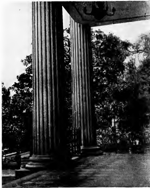
DETAIL—"STANTON HALL" PORCH
