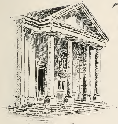
BATTERSEA CHURCH, WEST FRONT
