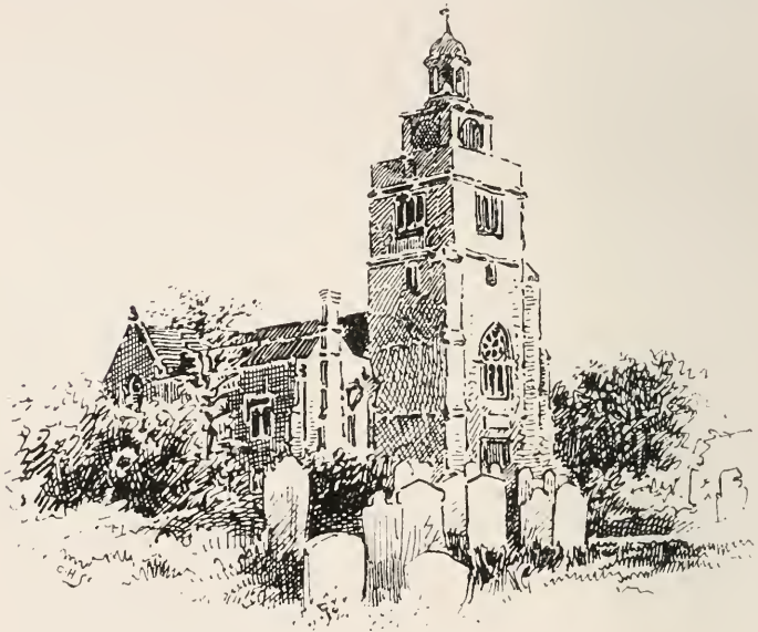
HAMMERSMITH OLD CHURCH (DEMOLISHED).
