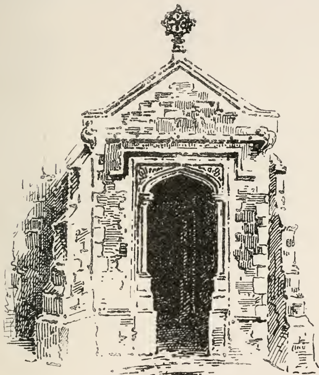
ST DUNSTAN, STEPNEY - SOUTH PORCH
