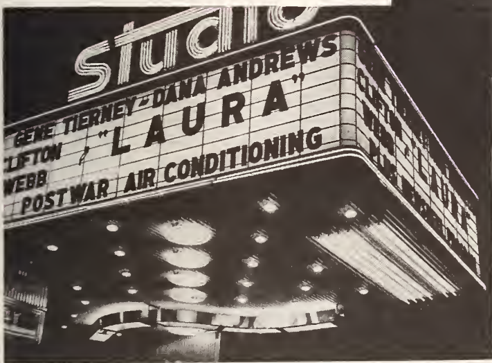
Floor plan of the Studio, cutting back behind valuable commercial space. The marquee is the principal identifying feature of the theatre front (right), the soffit of which (below) provides high illumination from neon rings and reflector lamps.
