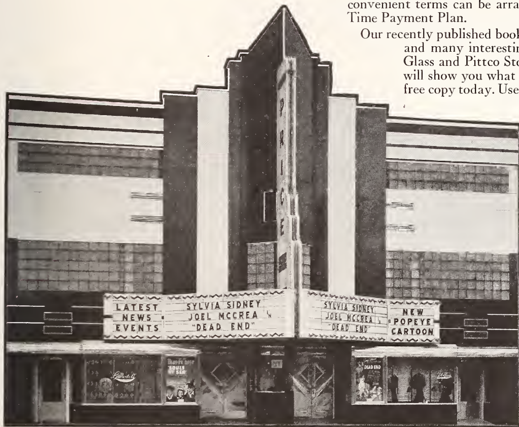
A MODERN THEATRE, like this one in Salt Lake City, Utah, has magnetism. It draws passers-by . . . invites them to enter . . . increases your profits. Follow this example by modernizing your theatre with Pittsburgh Glass and Pittco Store Front Metal. Architects: Ashworth & Markham.
