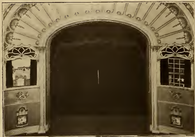
Stage of the Liberty, of Seattle, showing the interesting "boxes" on either side, from which were worked unique lighting and scenic effects.
