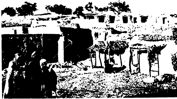
FIGURE 5. Most villages are constructed of closely spaced mud-brick or stone buildings; roofs generally are flat (U/OU)
