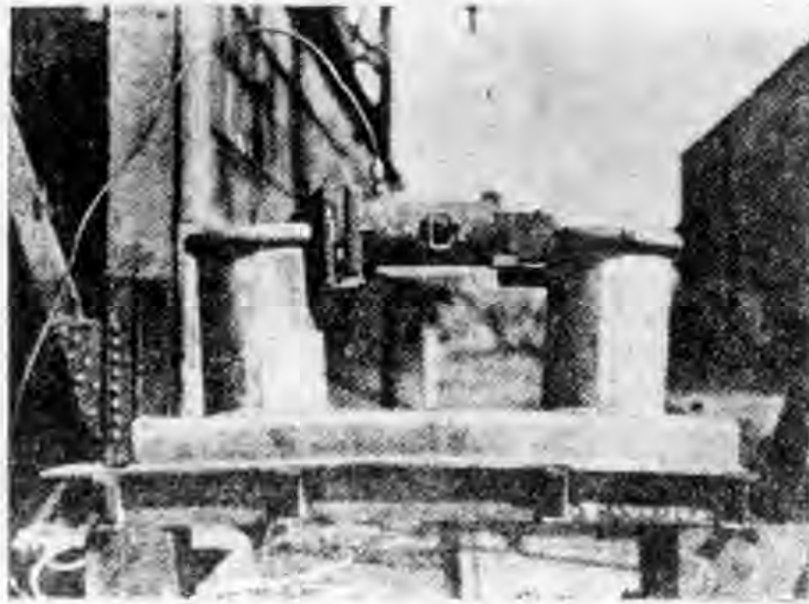
鑄接雙錨泊之繫船柱
