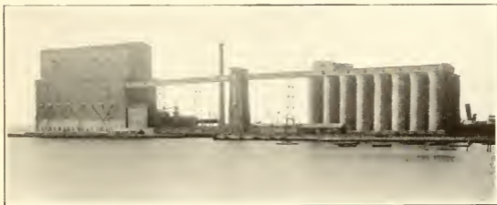
One of Baltimore's Great Grain Elevators
