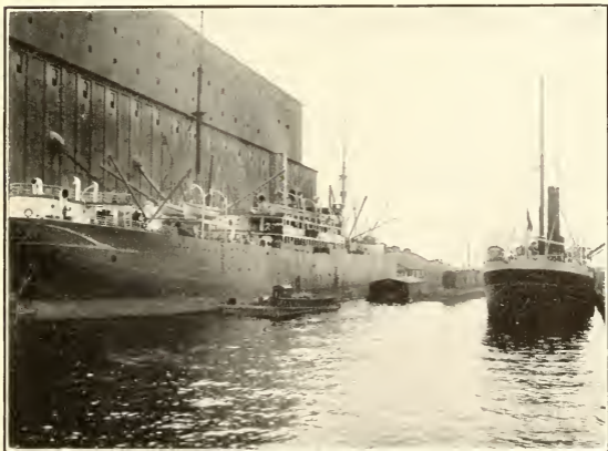
Great Piers of the Baltimore and Ohio Railroad
