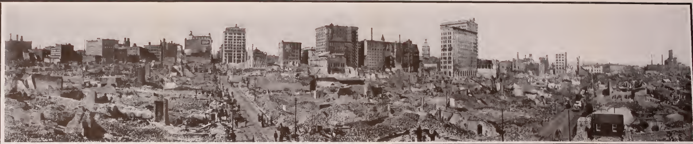
1904—February 7, 8, fire swept over 140 acres, destroying 86 blocks of buildings in the business center of Baltimore; loss $125,600,000. This picture is a partial view of the ruins
