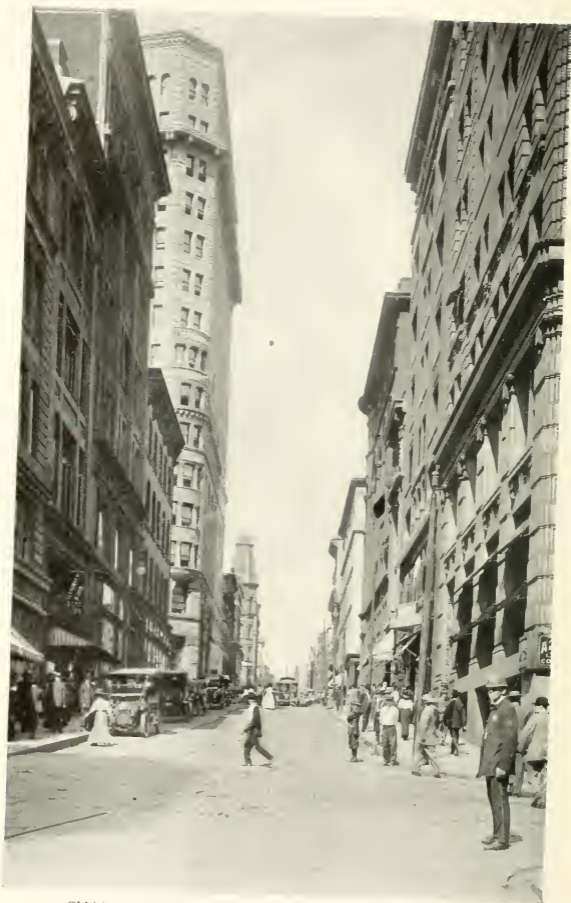
CHARLES STREET, NORTH FROM FAYETTE STREET
