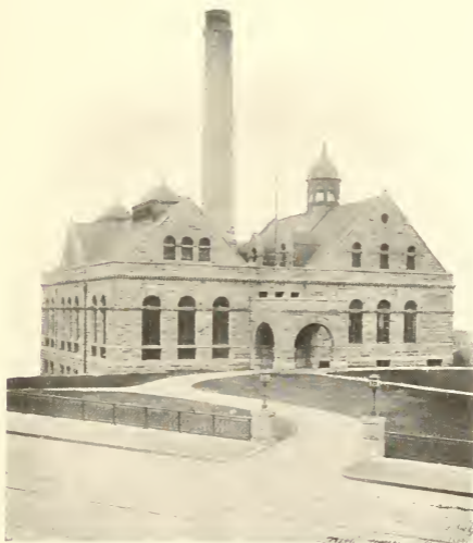
Baltimore's Water Supply—Mt. Royal Pumping Station
