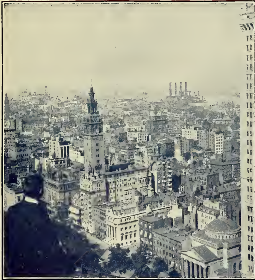
From Flatiron Building—Northeast, past Madison Square to Queensboro Bridge (Right)
