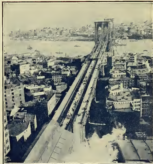
Brooklyn Bridge, New York Side
