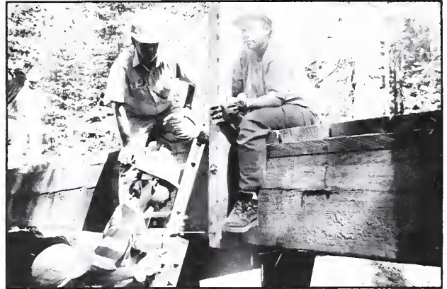
TASC students gain experience building a bridge
