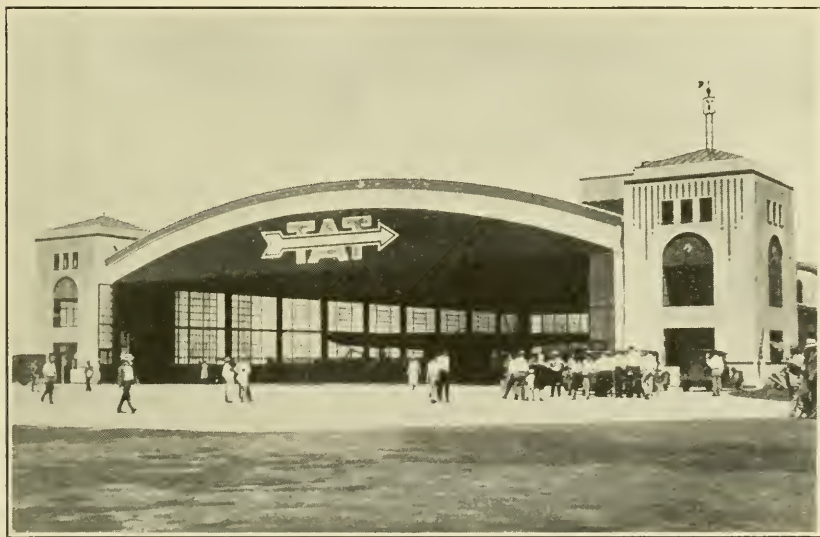
Front view of TAT hangar, Port Columbus, Ohio.
