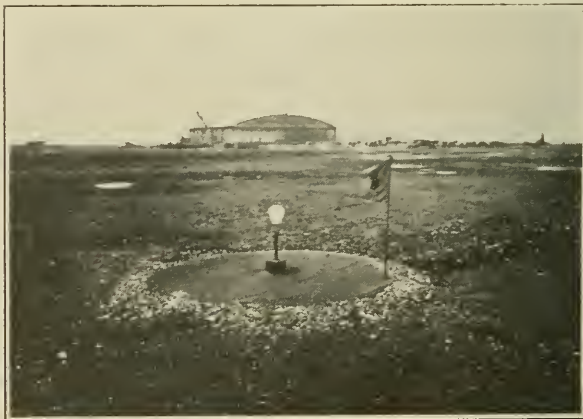
Boundry marker unit equipped with a 60-watt lamp. These units are spaced at less than 300-foot intervals on the boundaries of a landing field.
