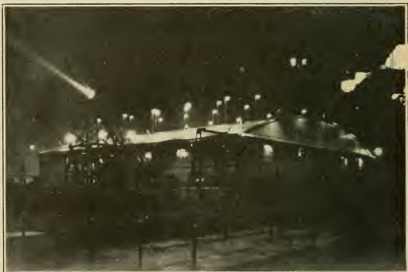
The exterior of this hangar is illuminated to an average intensity of 2\frac{1}{2} -foot candles by means of 200-watt lamps in industrial type reflectors.
