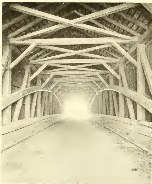
INTERIOR OF A COVERED TURNPIKE BRIDGE
