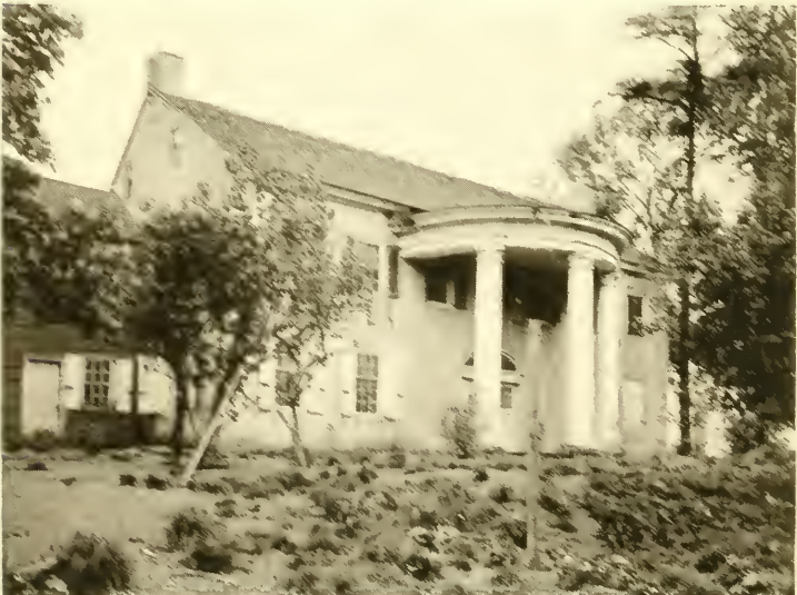
OLD FARM HOUSE, NEAR ABBEVILLE ROAD
