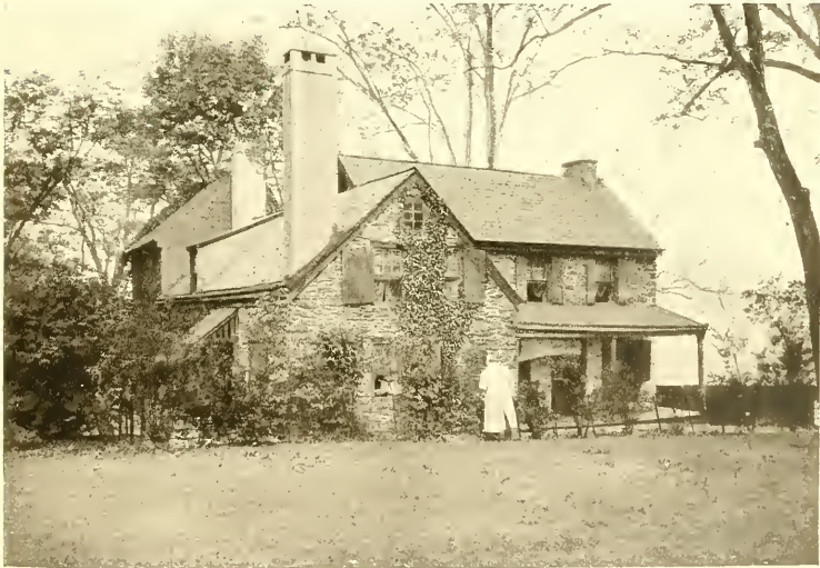
OLD FARM HOUSE Near the gate of Butler Place, the country home of Mr. Owen Wister
