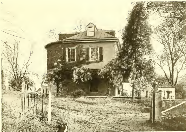
COMMODORE STEPHEN DECATUR HOUSE, POWDER MILL LANE, FRANKFORD
