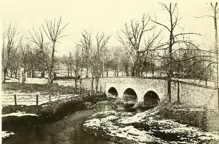
BRIDGE OVER THE POQUESSING AT TORRESDALE
