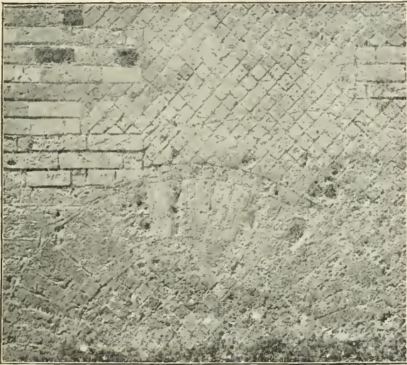
Fig. 12.—Reticulate facing, with corners of brick-shaped stone. The filled arch is probably to bear the weight of the wall over a sewer.
