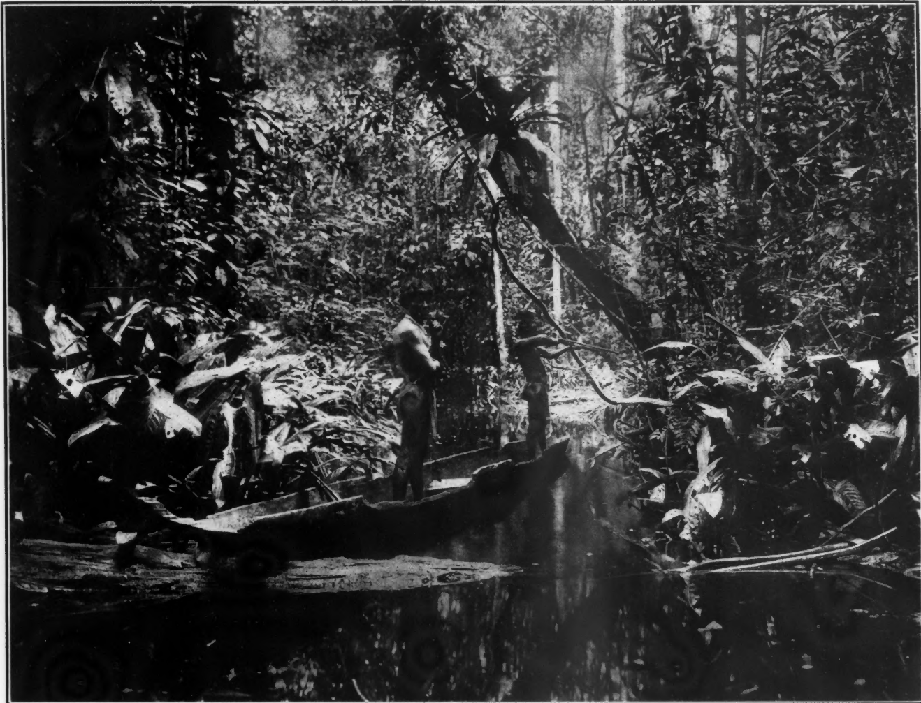
DREDGING GROUND IN THE TROPICS
