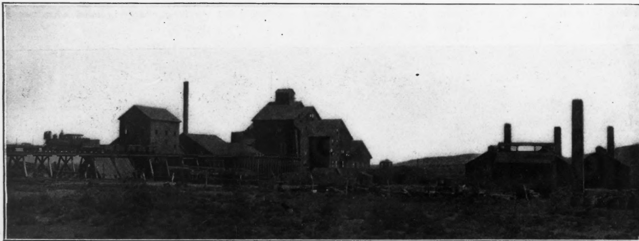
ADELAIDE REDUCTION WORKS, GOLCONDA, NEV.
