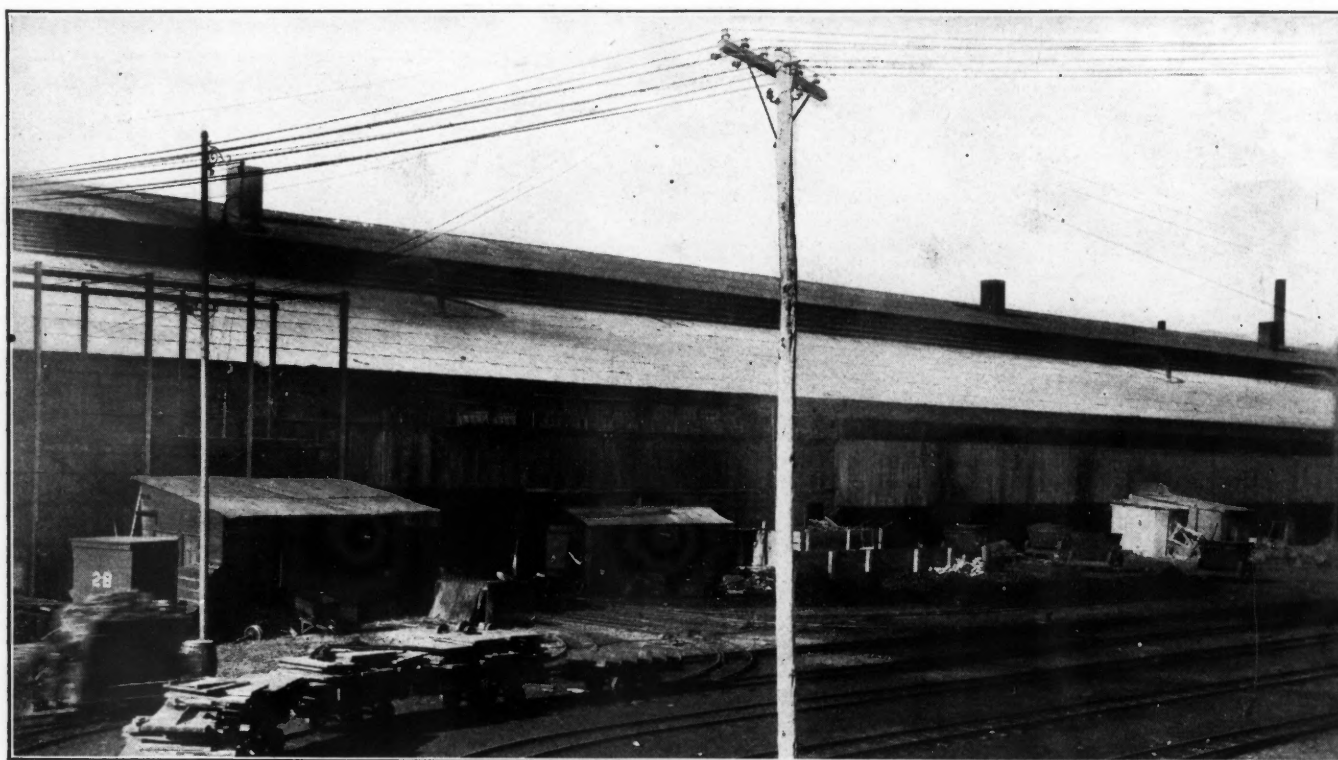
VIEW OF FURNACE BUILDING AT U. S. METALS REFINING CO.'S PLANT, CHROME, N. J.
