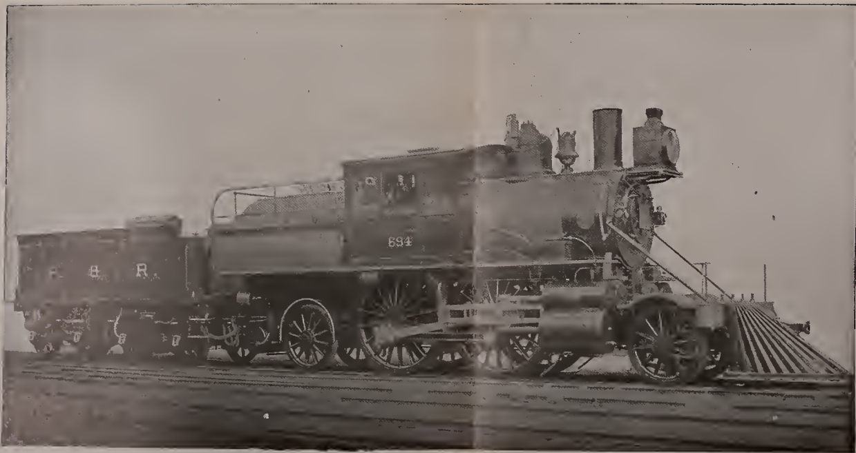
PLATE VII.—Compound Express Passenger Engine, No. 694, Philadelphia & Reading Railroad. Built by Baldwin Locomotive Works.
