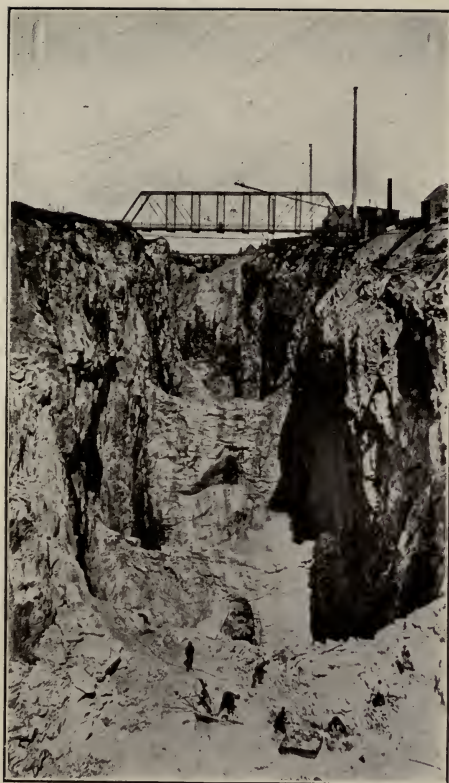
FIG. 1.—Limestone Quarry, Rockland, Maine. [From photograph by E. S. Bastin, U. S. Geological Survey.]
