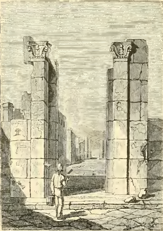
VIEW OF THE ENTRANCE TO THE HOUSE OF PANSA.
