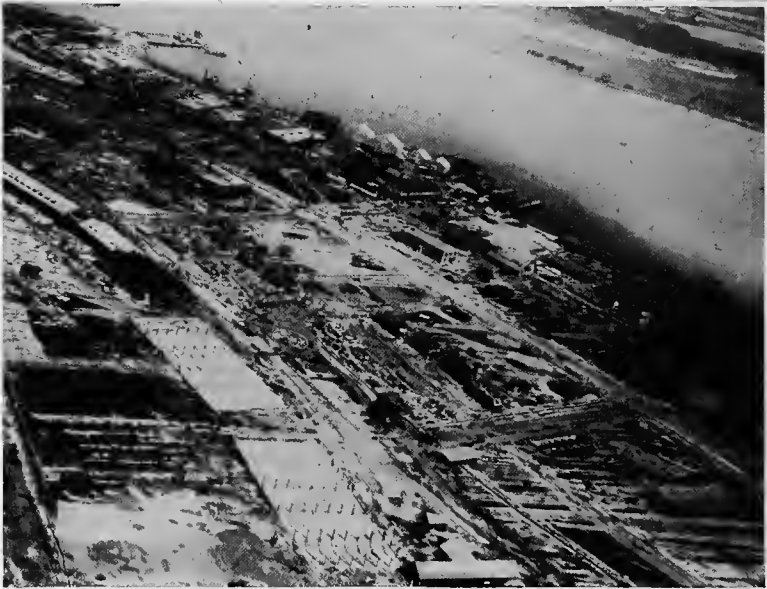
FIG. 196.—An aviation field under construction; early stage.
