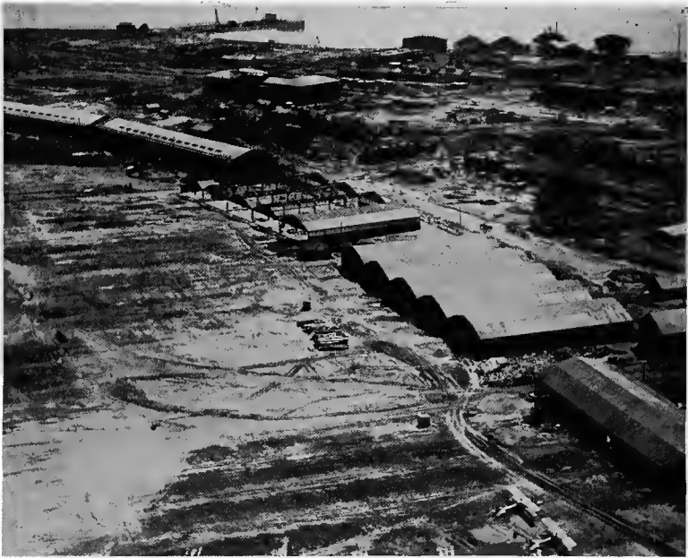
FIG. 197.—An aviation field under construction: later stage.
