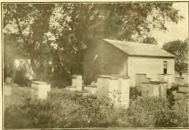
Honey house built in eight-foot sections to facilitate moving when necessary.
