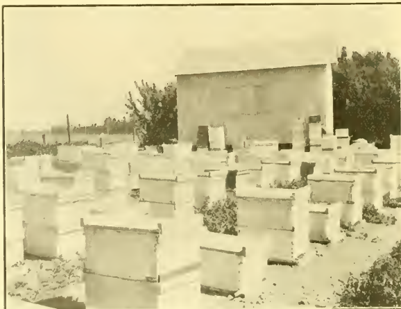
THE IRON FIRE PROOF EXTRACTING ROOM AND STOREHOUSE COMBINED AT THE FAR END OF THE GARDEN
