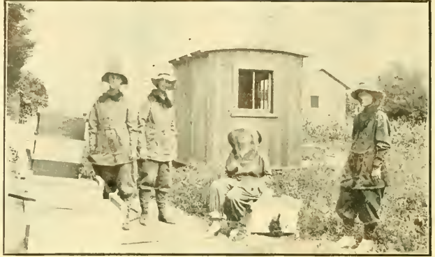
A crew of women workers at the Mendleson yards
