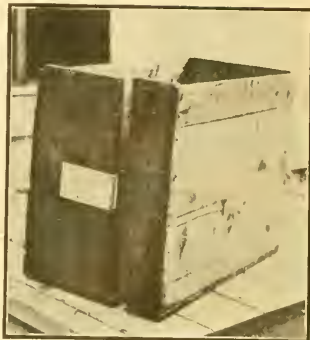
Ends without cleats are in danger of splitting.
