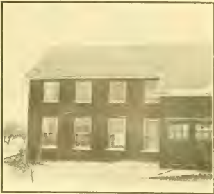
Rear view of Pettit Apiary Building
