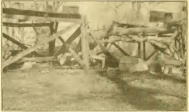
A sycamore fell during a storm and broke the trestle on which the apiary is kept above the river floods. Photograph by Winfield Gear.
