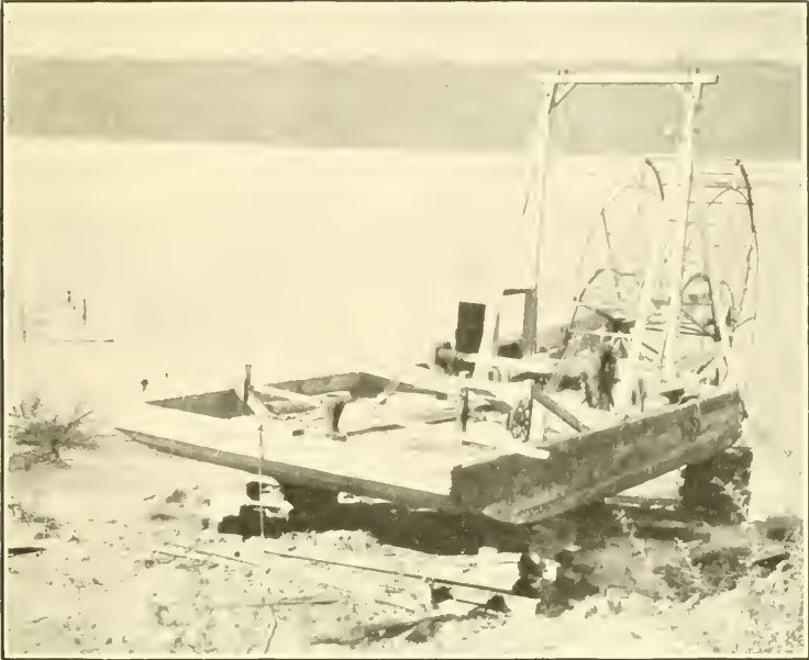
FIG. 23.—A COLUMBIA RIVER SCOW FISH WHEEL.
