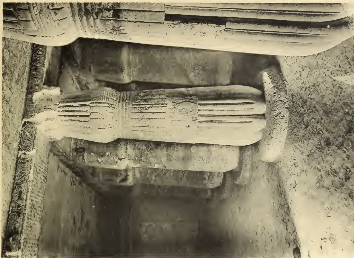
THE HALL. LOOKING EAST.
