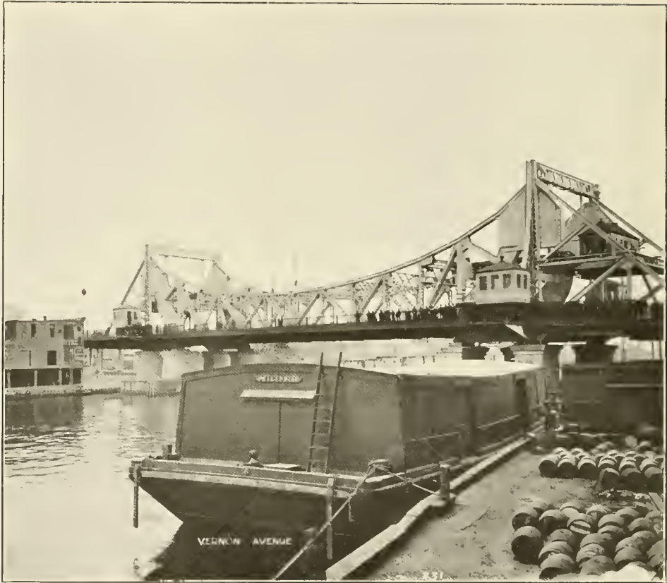
VERNON AVENUE BRIDGE OVER NEWTOWN CREEK.
