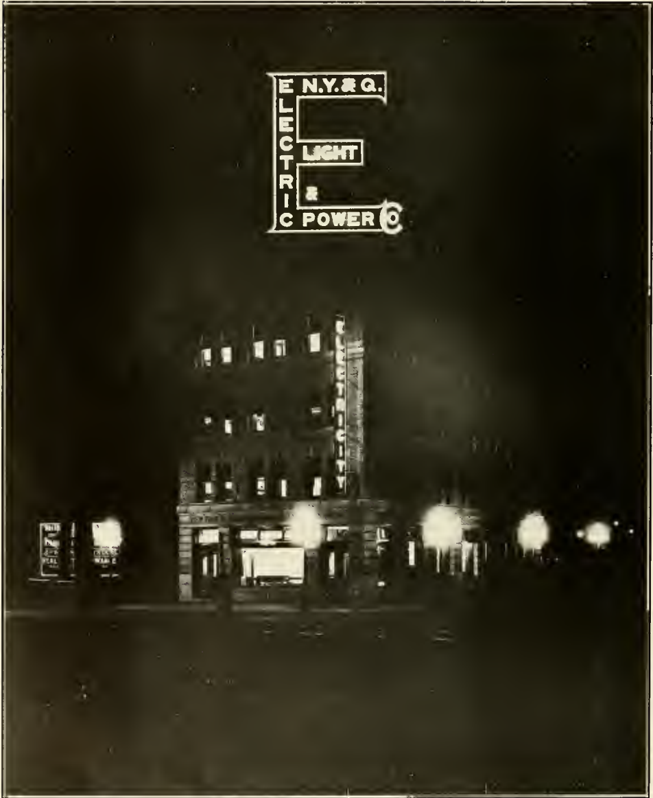
NIGHT VIEW OF BUILDING OF NEW YORK AND QUEENS ELECTRIC LIGHT AND POWER CO., QUEENSBORO BRIDGE PLAZA.
