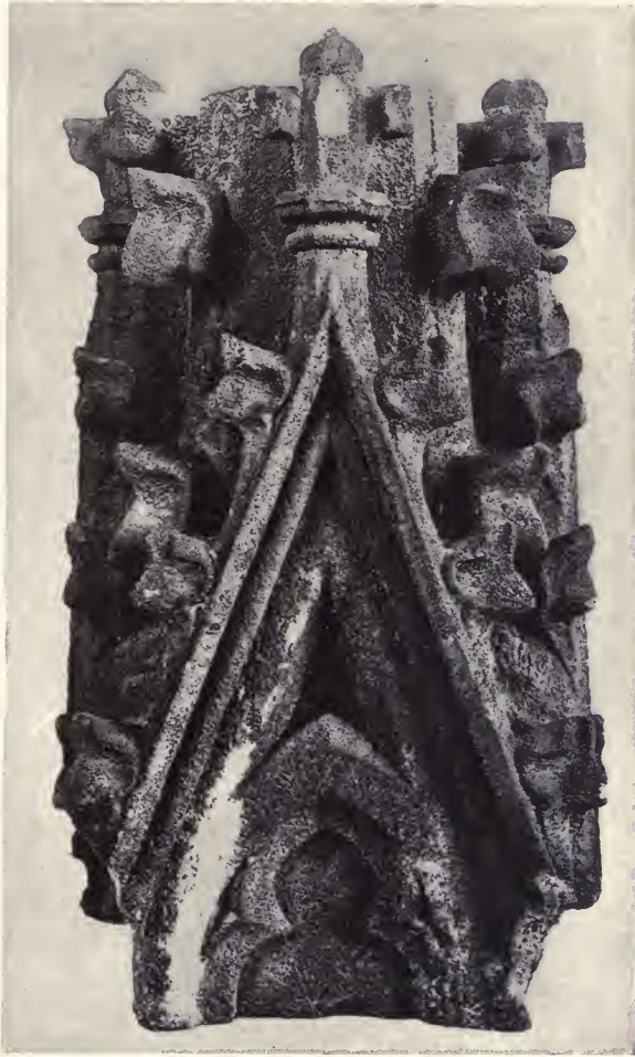
PLATE XVIII. — Scum of soluble salts, which has caused surface disintegration of sandstone. (After Kaiser, Neues Jahrb. Min., 1907, II.)
