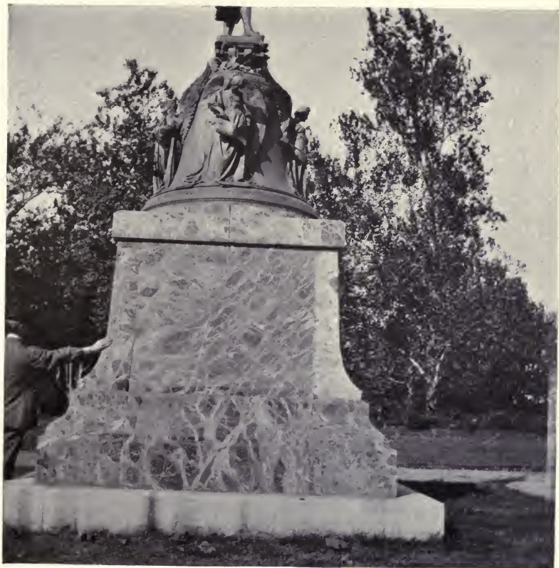
PLATE XLIII.—Serpentine Pedestal, Charlottesville, Va. This stone has been attacked to an appreciable extent by the weathering agents. (Photo by H. Ries.)
