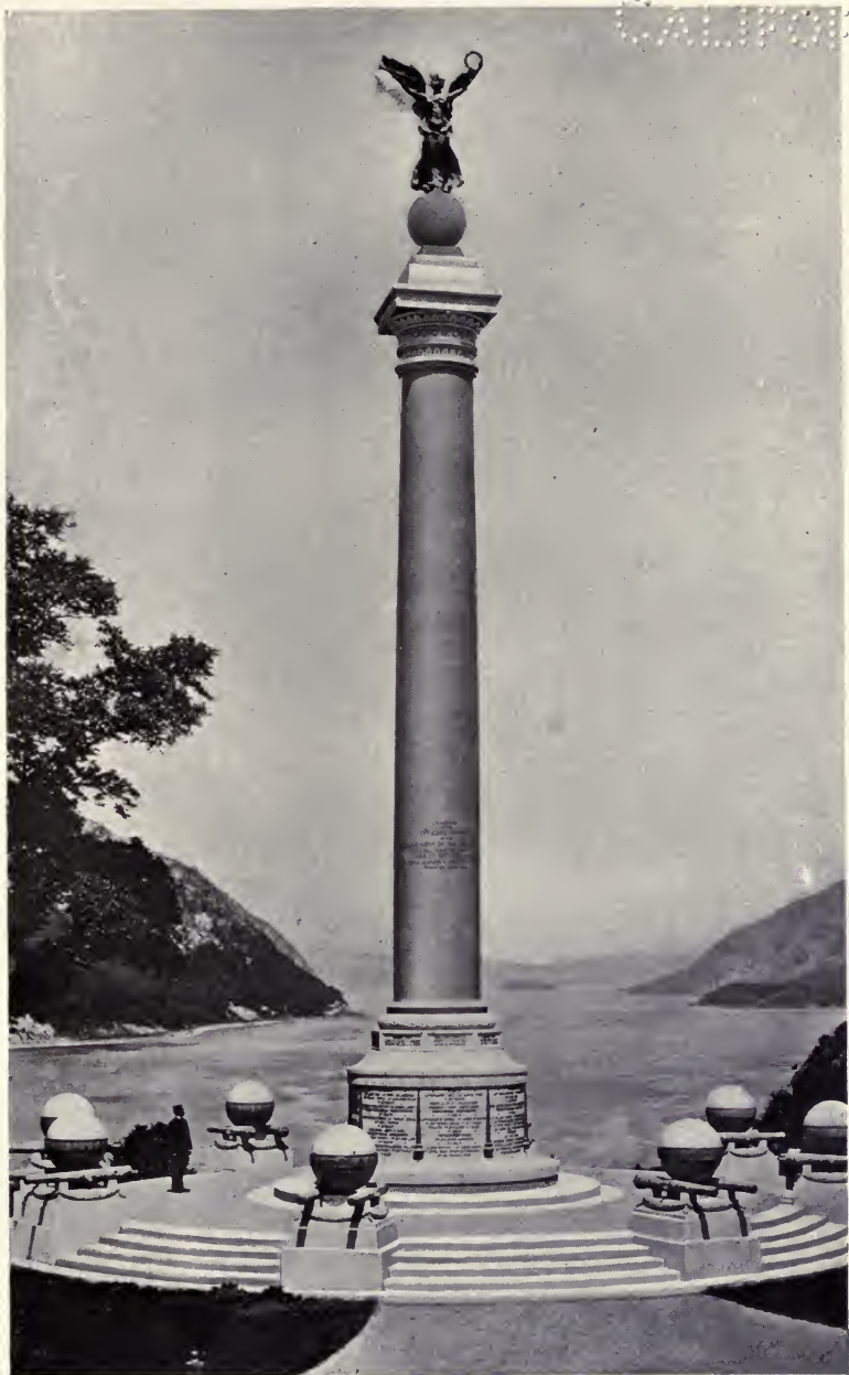
PLATE XXVI.—Battle Monument, West Point, N. Y. Polished shaft of Branford granite, 41 feet 6 inches long and 6 feet in diameter. (Photo loaned by Norcross Bros.)
