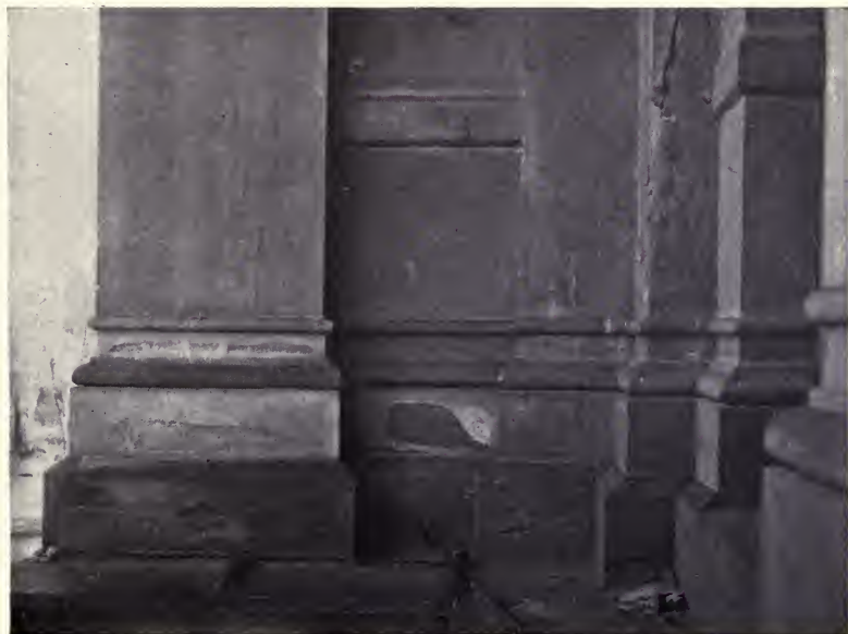
PLATE XVII, Fig. 2. — Weathered sandstone, second story, County Court House, Denver, Colo. (Photo by R. D. George.)
