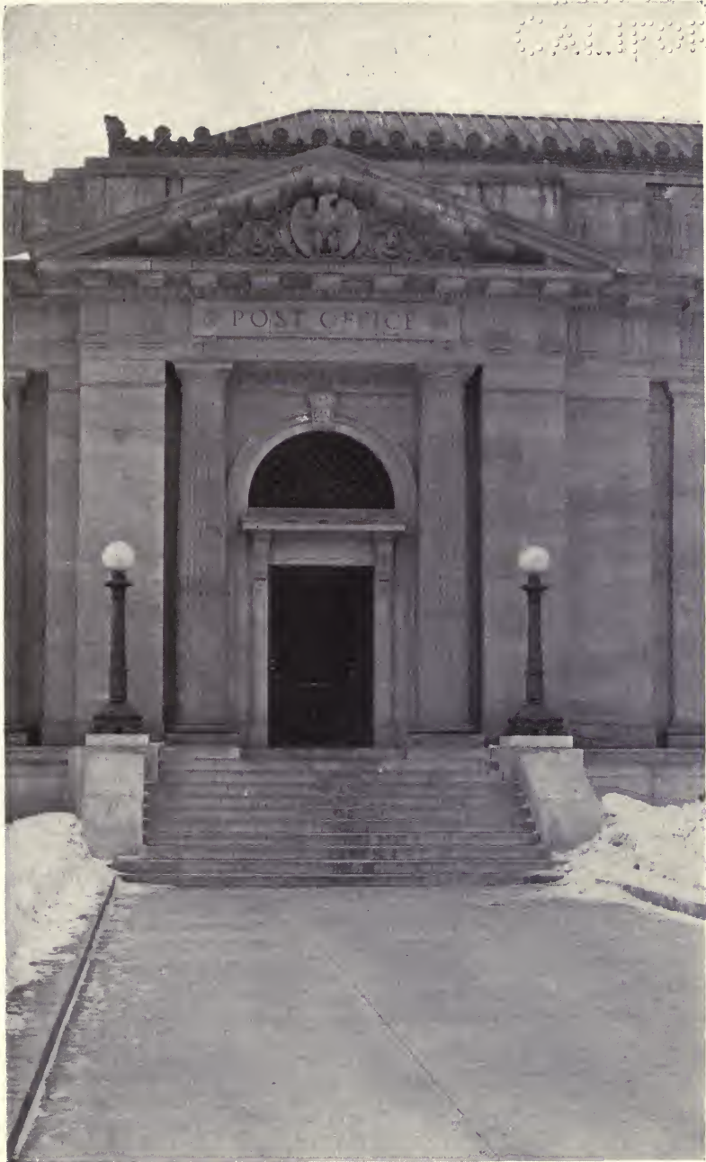
PLATE XXX. — U. S. Post Office, Toledo, Ohio, constructed of Gay "Canyon" Berea sandstone. (Photo loaned by Cleveland Stone Co.)
