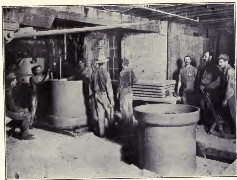
PLATE LVII, Fig. 2. — Molding 30-inch sewer pipe in pipe press.
