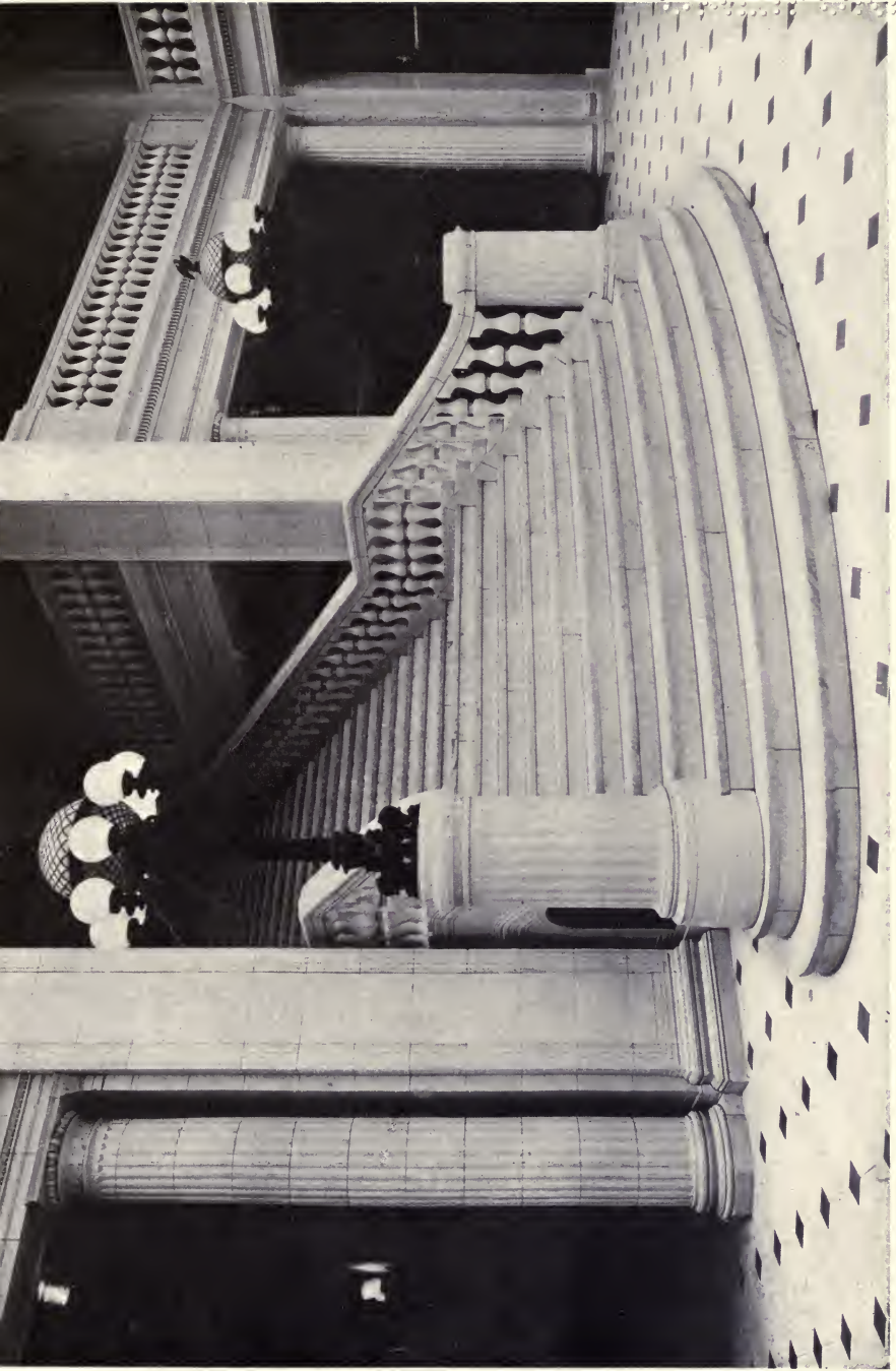
PLATE LIV. — Interior of Railway Exchange Building, Chicago, Ill. All glazed terra cotta except steps and floor which are marble. (Photo from Northwestern Terra Cotta Company.)
