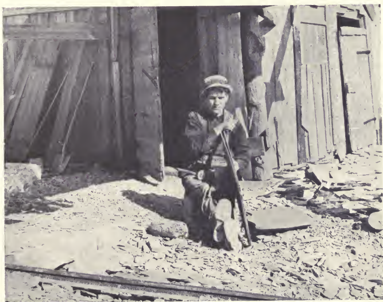
PLATE XLI, Fig. 2. — Splitting slate. (Photo by H. Ries.)
