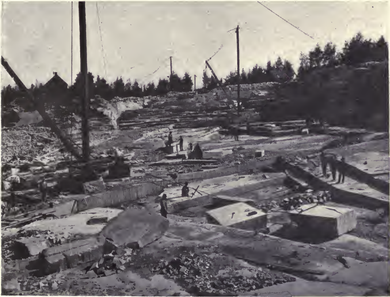
PLATE XX, Fig. 2. — Granite quarry at North Jay, Me. (Photo loaned by Maine and New Hampshire Granite Company.)
