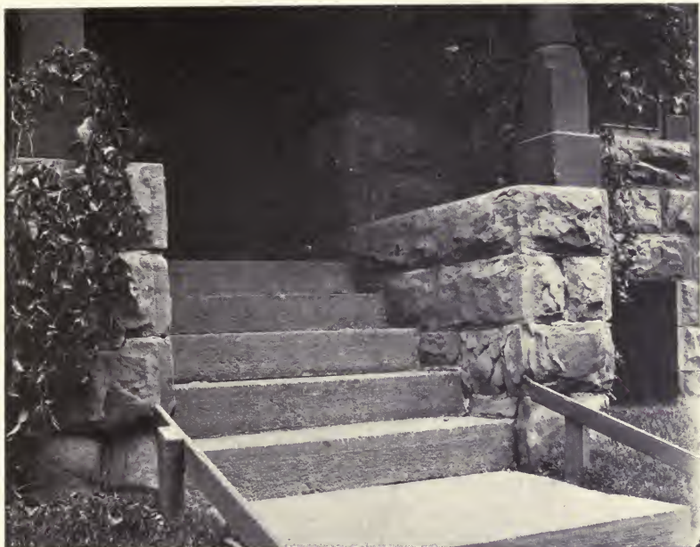
PLATE XVII, Fig. 1. — Weathering of red sandstone, Denver, Colo. (Photo by R. D. George.)
