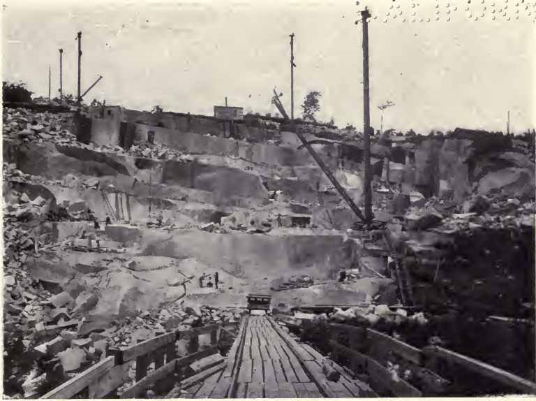
PLATE XX, Fig. 1. — Granite quarry, Hardwick, Vt.
