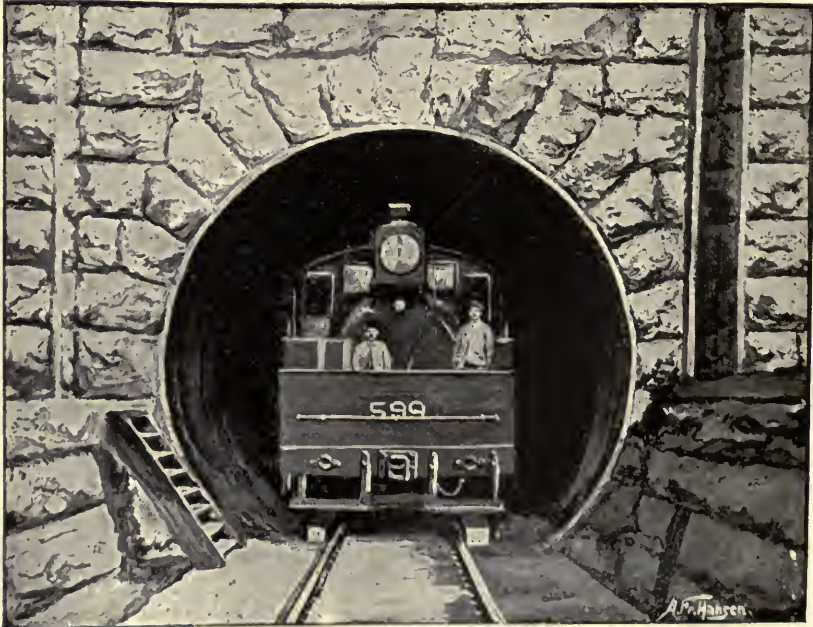
TUNNEL ENGINE EMERGING FROM PORTAL.
