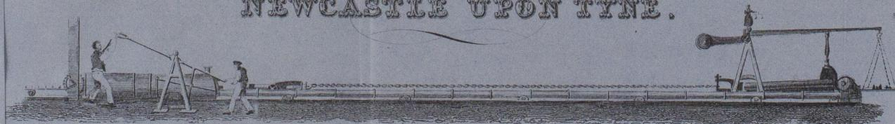
TESTING MACHINE FOR PROVING CHAIN CABLES
