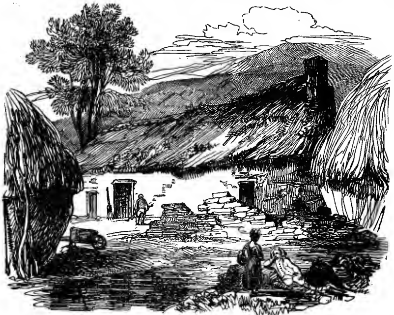
MUIRHOUSE, EAGLESHAM, RENFREWSHIRE :
