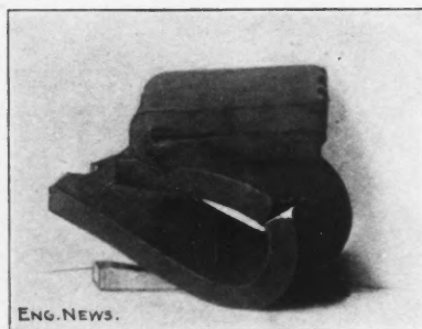
Bending Tests of Steel Plates.
