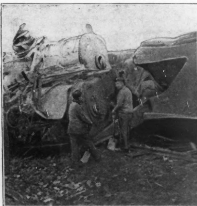
Fig. 4.—View from the Rear. (The boiler on top was turned completely around.)
