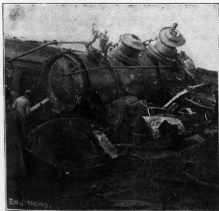
Fig. 3.—View From the Front, Showing Least Injured Boiler.
