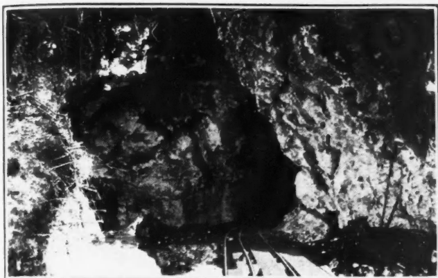
Entrance to drift, showing magnesite on both sides
