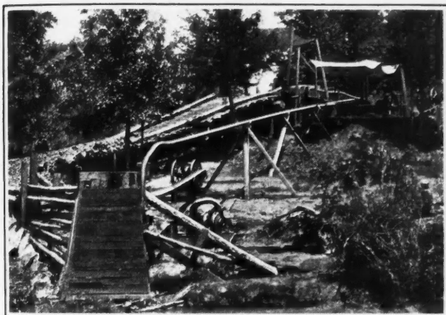
Crude washer at Roach mine
