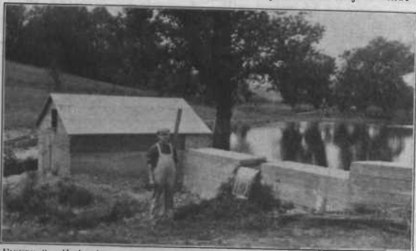
FIGURE 3.—Hydroelectric plant built in Pennsylvania in 1925. Drainage area 2.4 square miles, head 6.9 feet, steel overshot wheel 6 by 2½ feet, generator one-half kilowatt, power house 13 by 15 feet. Cost of machinery $385, materials $325, labor $356, wire $64, miscellaneous $128, total $1,258. Estimated cost of current, including interest, depreciation, taxes, insurance, attention, and repairs, $174 per year
