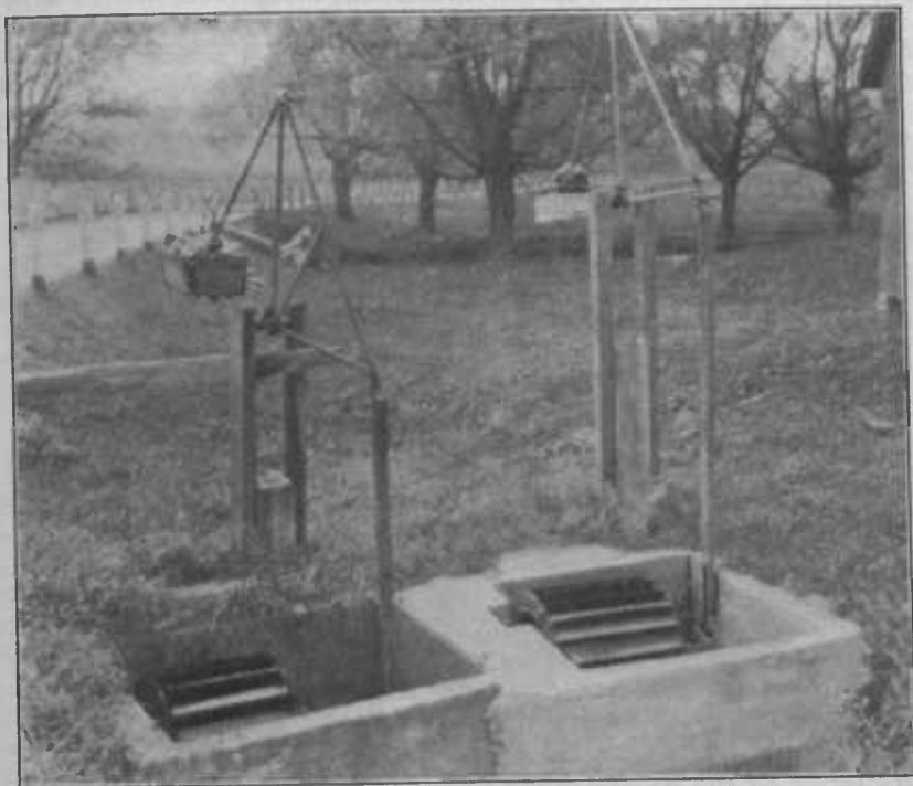
FIGURE 18.—Two pitch-back wheels, in Pennsylvania, which make about six revolutions per minute and are connected by 8-inch cranks (16-inch stroke) to counter-weighted steel triangles having draft wires to two pumps about 400 feet away. The left wheel cost $45 at the shop 15 years ago and the right wheel cost $75 recently.
