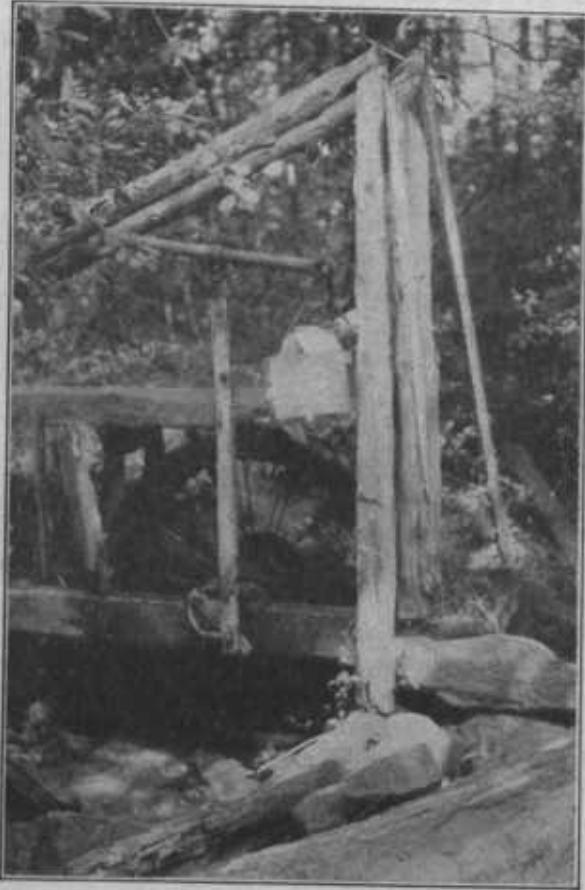
FIGURE 1.—Inexpensive overshot wheel and homemade counterweight rocker arm with draft wire for transmitting the power. Virginia
