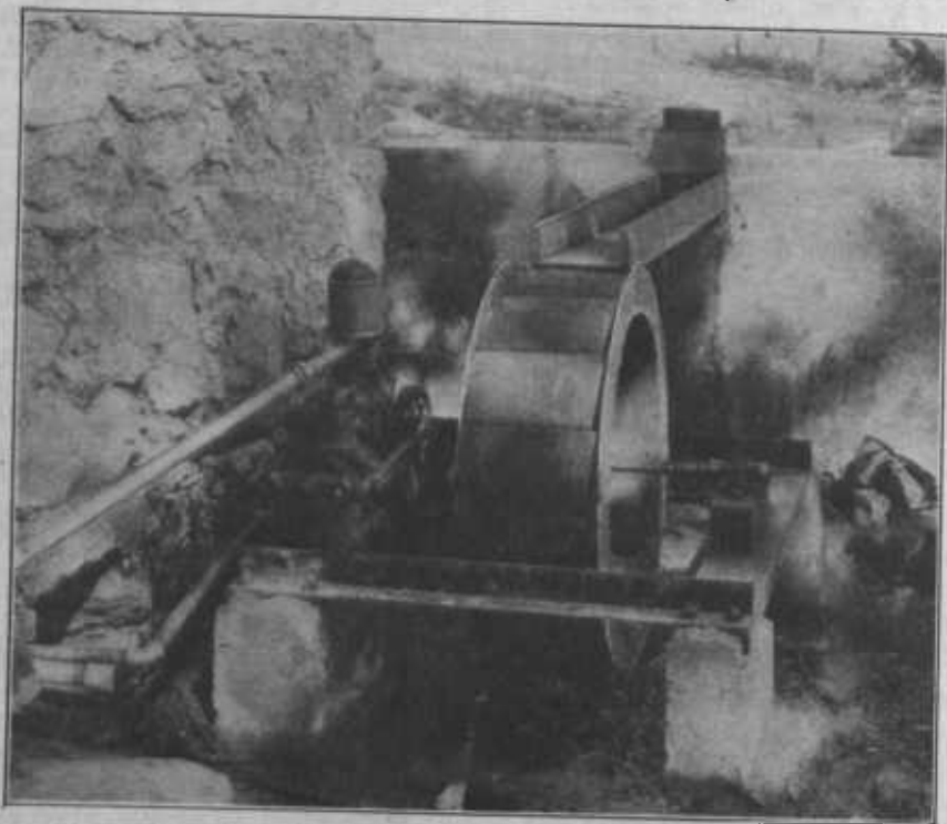
FIGURE 13.—Faulty application of water to a small (3 by 1 foot) steel overshot wheel installed in Virginia in 1915. Cost of wheel, shaft, and gear, $60; shop-made steel frame and two pillow blocks, $35; 2\frac{1}{2} by 4 inch pump, $60
