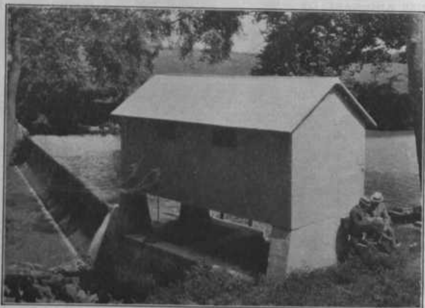
FIGURE 7.—Mutually owned plant built on the site of an old timber dam. Power house 8.6 by 20 feet, concrete dam 141 feet long, drainage area 51 square miles, head 7.5 feet. Cost of 27-inch turbine $393, 6-kilowatt generator $550, governor $460, materials $1,582, labor $1,000, wire $632, rent and supplies $250, instruments and miscellaneous $821, total $5,688. Approximately two-thirds of the cost was for the dam. Estimated cost of current per year, $754
