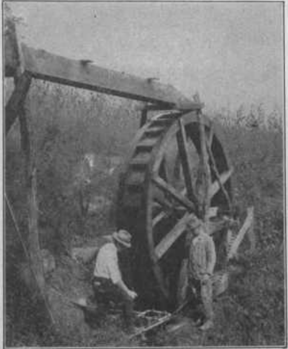
FIGURE 2.—Simple wooden flume and overshot wheel with chain drive to a pump lifting spring water to a mountain home. North Carolina
