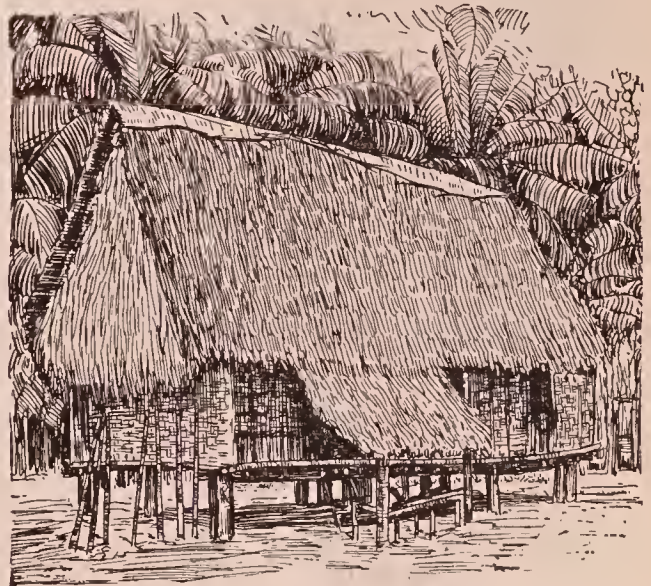
Guam native dwelling made of reeds and bamboo with roof of cocoanut thatch.
