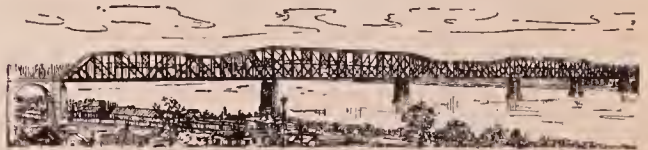
Cantilever Bridge over the Mississippi River at Thebes, Illinois.
