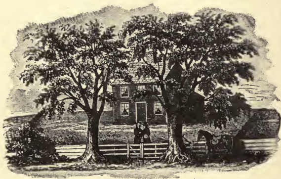
THE OLD JONATHAN EDWARDS HOUSE, NORTHAMPTON.
