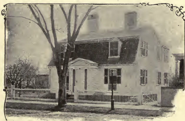
HAWTHORNE'S DEARBORN STREET HOUSE.
