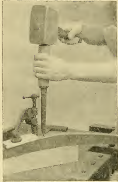
1. Mortising Leg on Saddle.
