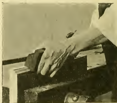
5. Using a Moulding Plane.
