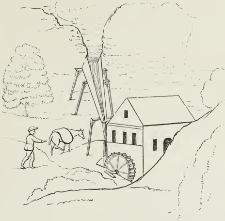
MILL, WITH SLUICE AND OVERSHOT WHEEL. Quintus Curtius, 46.
