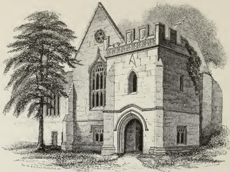
PORCH AND WINDOW OF THE CHAPEL.
