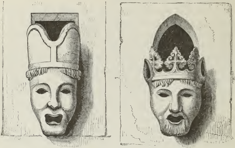
Openings in the Hall, Great Chalfield.
