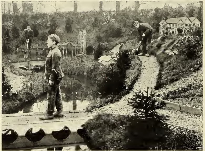
IRON-AND-CEMENT BRIDGE BUILT BY THE BOYS.
