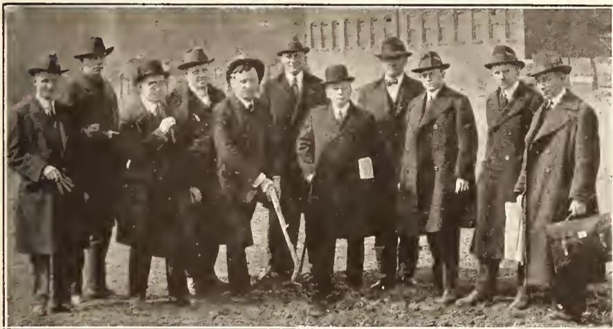
Messrs. Meisselbach, A. Heineman and Architect Corey With Meisselbach Factory Heads Breaking Ground for New Plant
