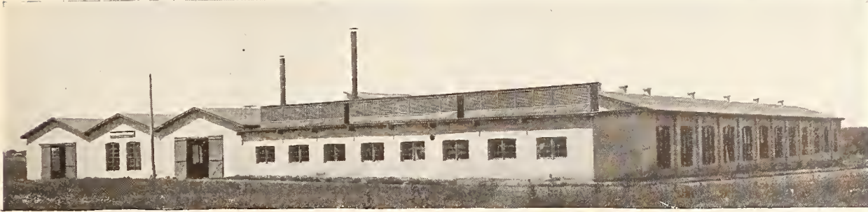
Plant of the Schwartz-Herrman Steel Works, Inc., Somerville, N. J.
