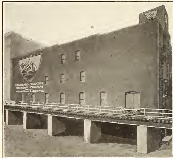
View of Private Railroad Siding
