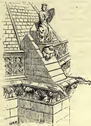
Amortizement of Buttress (13th century), Apsidal Chapel, Cathedral of Amiens.
